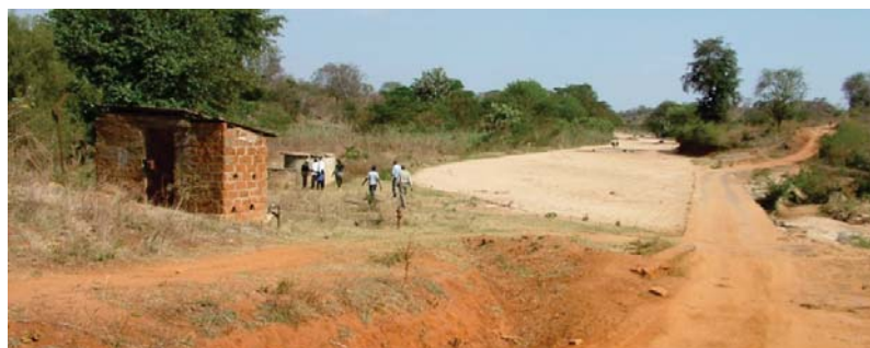
Figure 12. A sand dam road crossing between Kako and Kyaluma villages, Mbooni East sub-district, Makueni County, Kenya including shallow well and pump house
