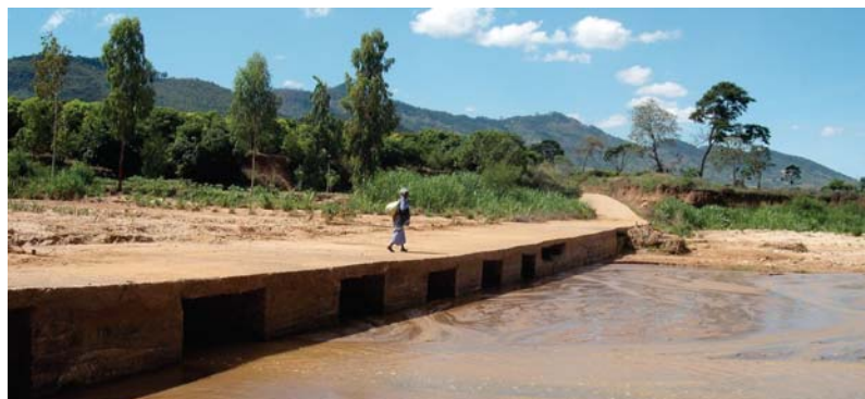
Figure 17. Dam 4, 200 m repaired and adapted culvert
