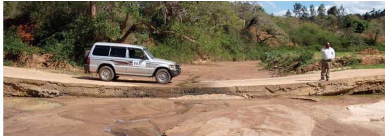
Figure 15. Dam 2, a small 24 m length drift
