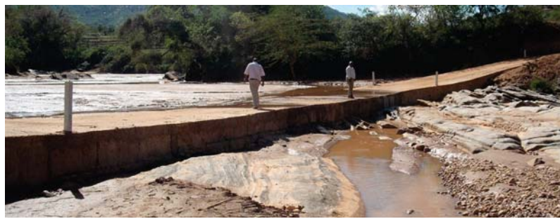
Figure 16. Dam 3, 80 m drift, built on bedrock
