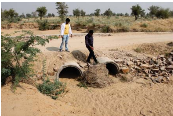
Figure 6. A failed culvert river crossing. A combination of insufficient flood capacity, poor headwall construction and unpaved road surface caused this culvert in India to fail. The river eroded a new channel to the left-hand side of this culvert
