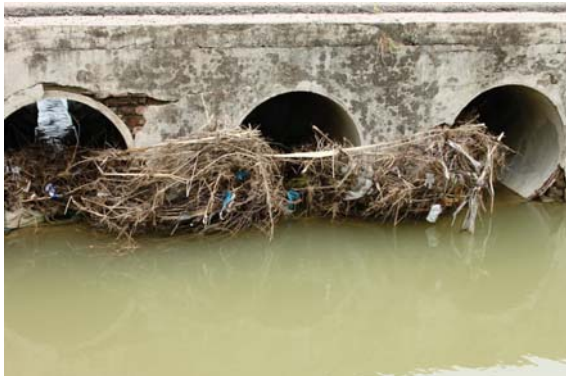
Figure 5. A restricted culvert in India: without regular maintenance to remove sediment and flotsam, the capacity of a culvert is greatly reduced
