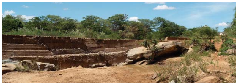
Figure 13. The view from below the dam shown in Figure 12. The spillway is 80 m wide, 1 m high and 2.5 m above the river bed
