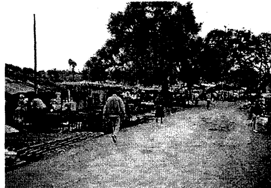
Urban road space often serves pedestrians and roadside stalls in addition to motorized traffic
