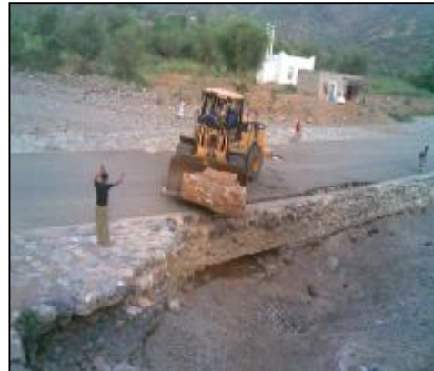
Figure 11. Damages to Irish Crossing Outlet in an Asphaltic Road
