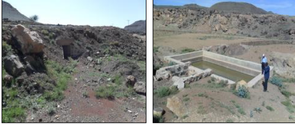
Figure 6. Water Harvesting Tanks from Culvert Outlet
