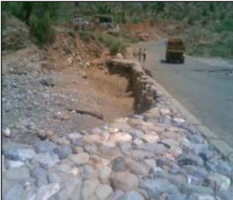
Figure 11. Damages to Irish Crossing Outlet in an Asphaltic Road
