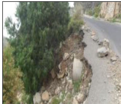
Figure 12. Damages to Box & Pipe Culverts in an Asphaltic Road
