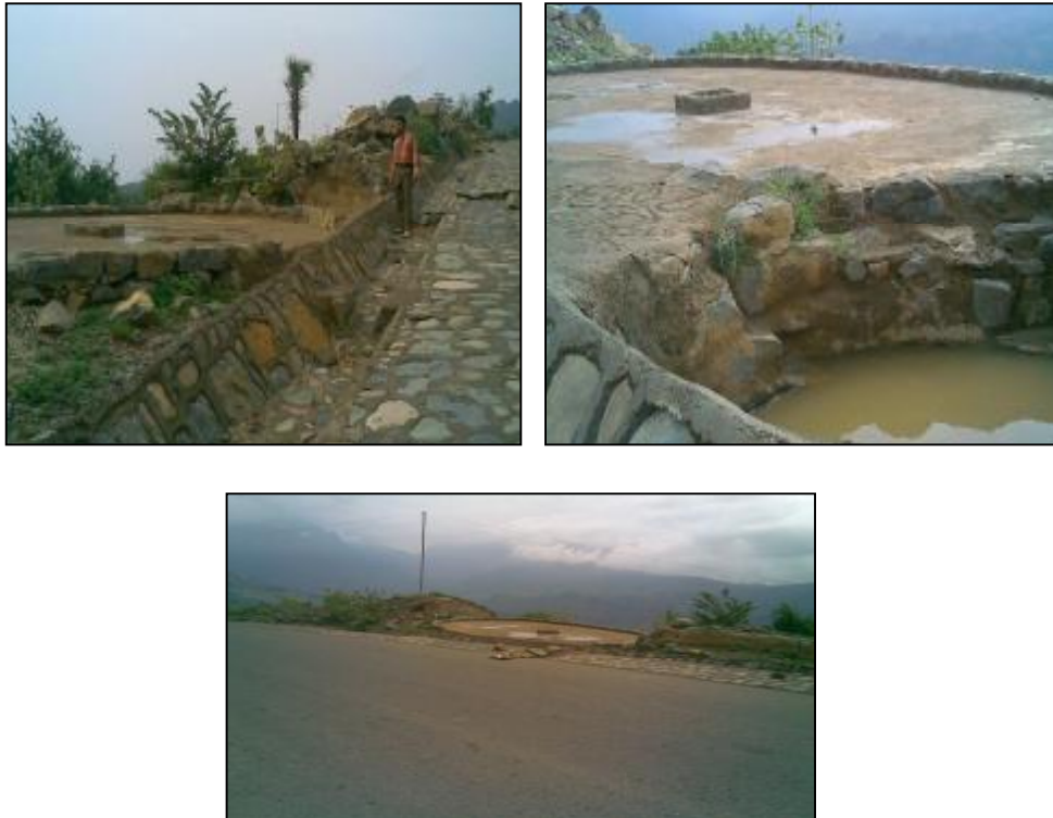
Figure 7. Water Harvesting Cistern from Side Ditches
