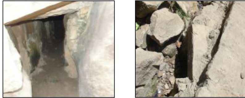
Figure 2 . Canal under Stone Paving
