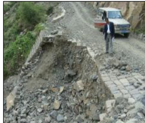
Figure 12-a. Damages to Irish Crossing Dry Stone Wall in Stone Paved Rural Road
