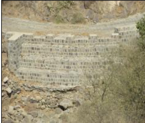
Figure 12. Damages to Irish Crossing Wall in Stone Paved Rural Road
