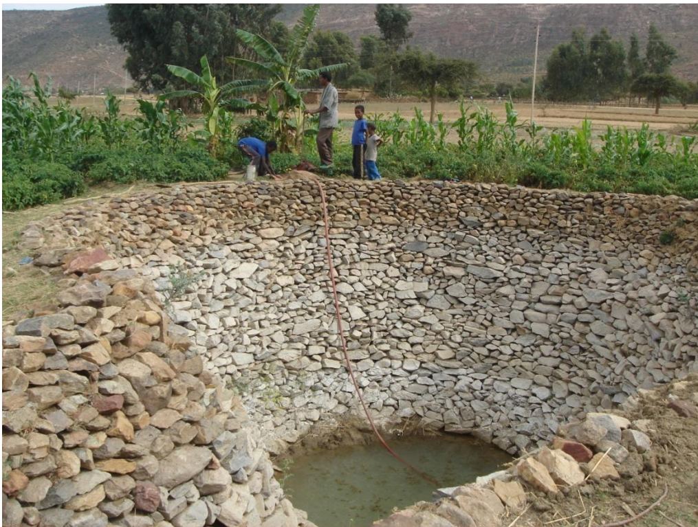
Plate 2b. Hand-dug well for small-scale irrigation along the Abreha Westbeha-Hawzien road.
