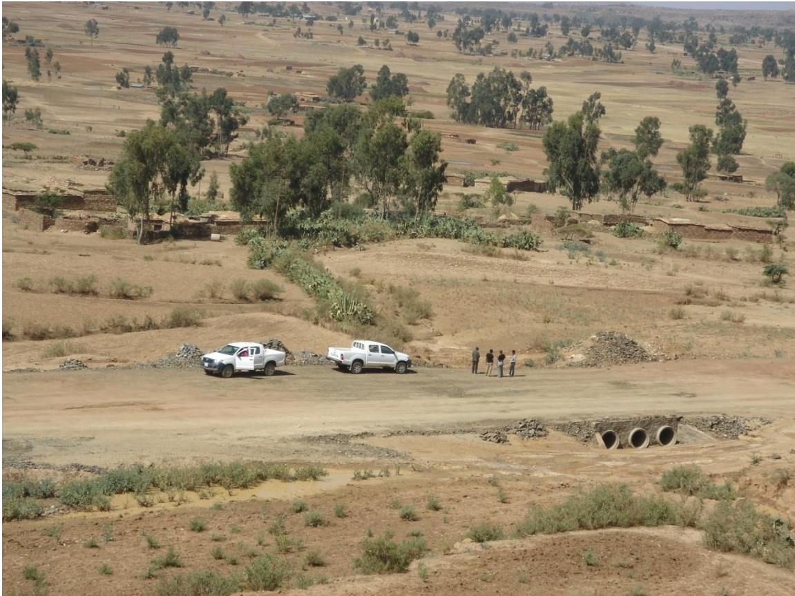
Plate 5: Ponding of water at the road side and endangered dwelling houses from floods from culverts. The consultant of the road plans to channel the flow from culverts down up to 1km from the road.
