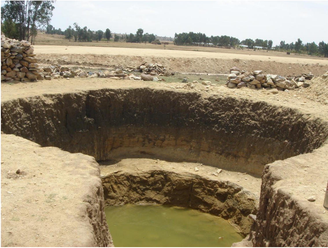
Plate 2a: A road passing close to an existing hand-dug well which is used for small-scale irrigation along the Freweign-Hawzien road.
