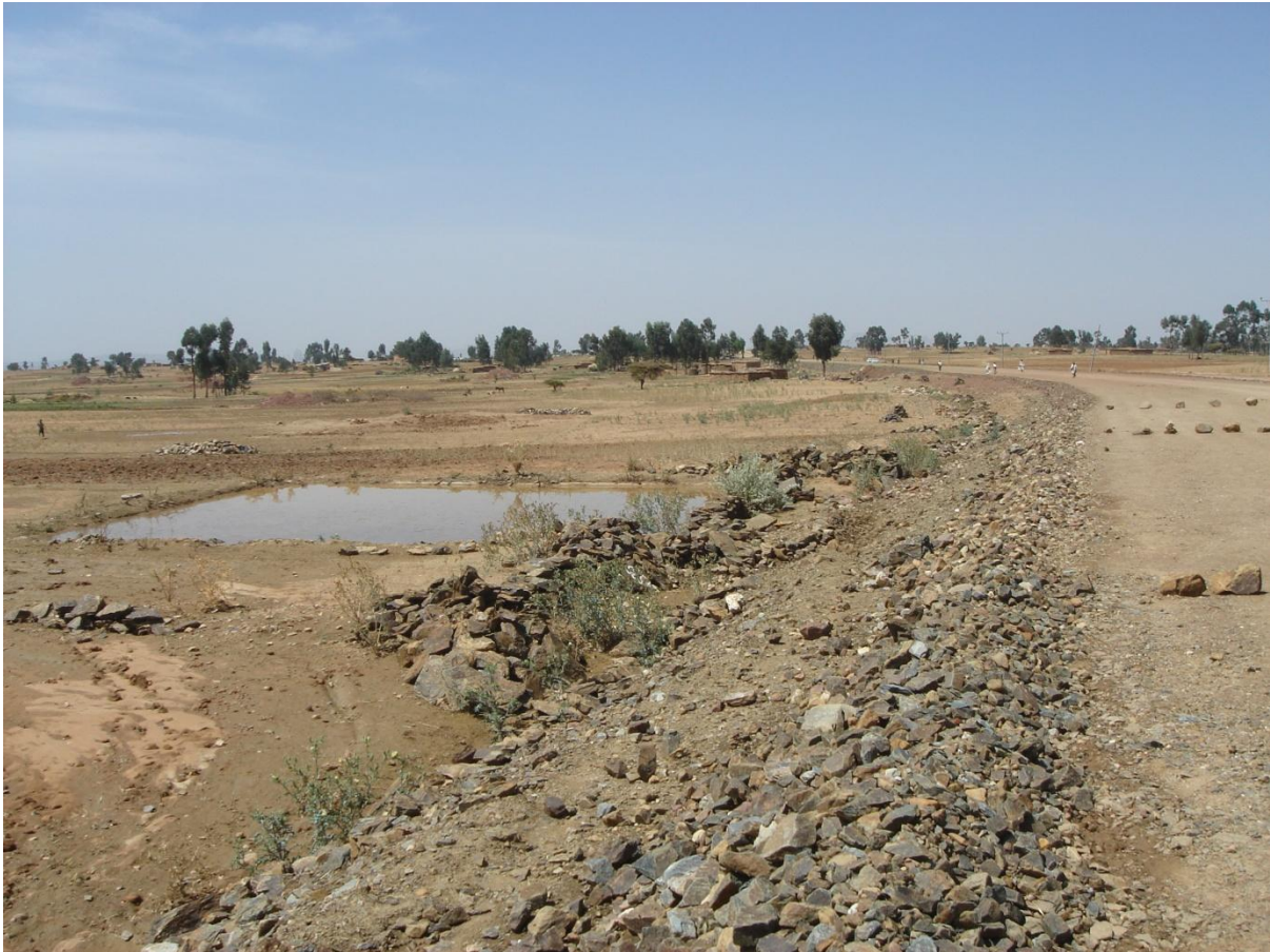
Plate 7: A 3m deep surface reservoir (Horeye) filled with flood water from road sides at the Freweign-Hawzien road.
