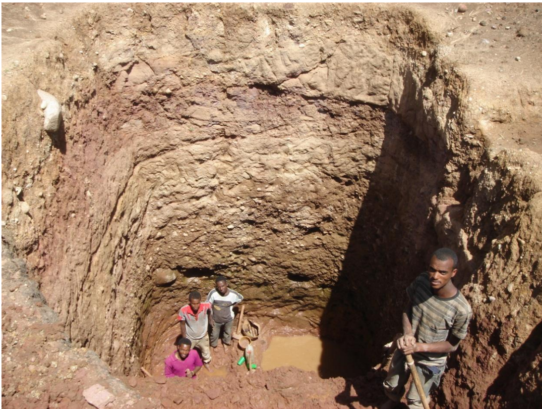
Plate 3: Hand-dug well which is under construction in Freweign (Sinkata) area .
