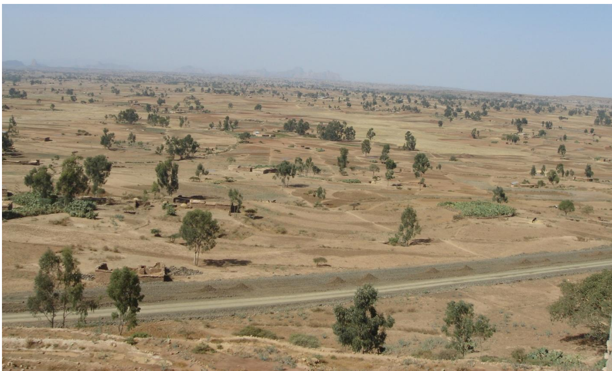
Plate 1: View of the plains at Freweign area which the road under construction passes through. The communities at down side of the road are endangered by the flood from culverts.
