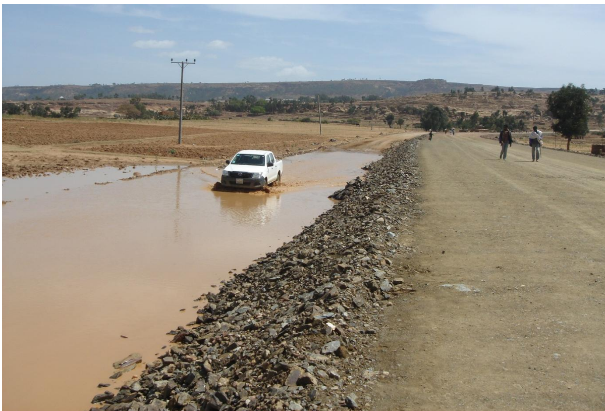
Plate 4: Ponding of water at the road side of the Freweign-Hawzien road.
