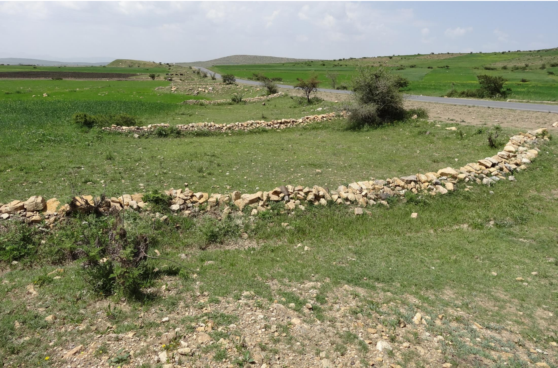
Plate 26. Road side runoff is diverted and spread into farm lands through series of channels, Tigray, Northern Ethiopia
