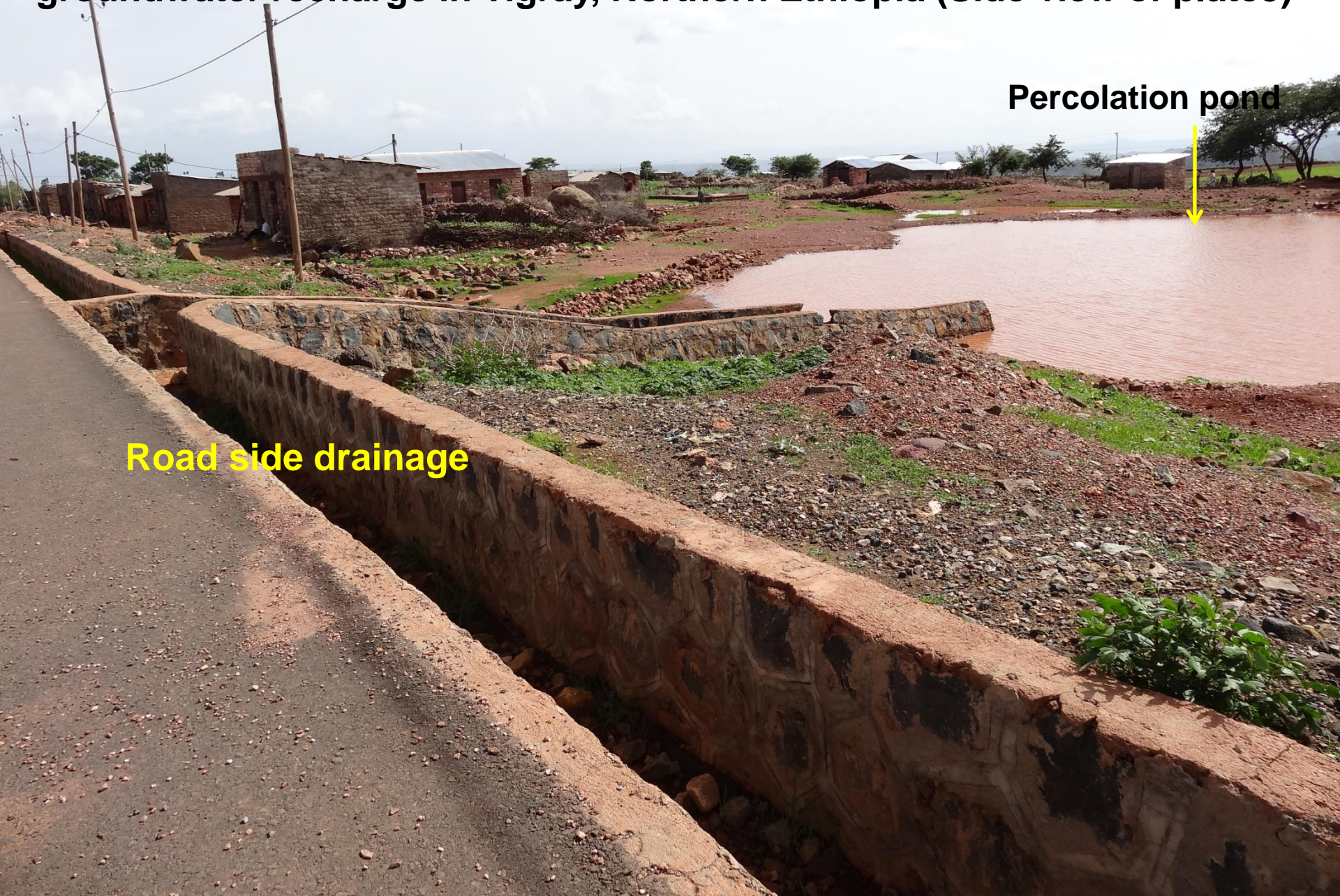
Plate 6: Road side drainage connected to percolation pond for groundwater recharge in Tigray, Northern Ethiopia (Side view of plate5)
