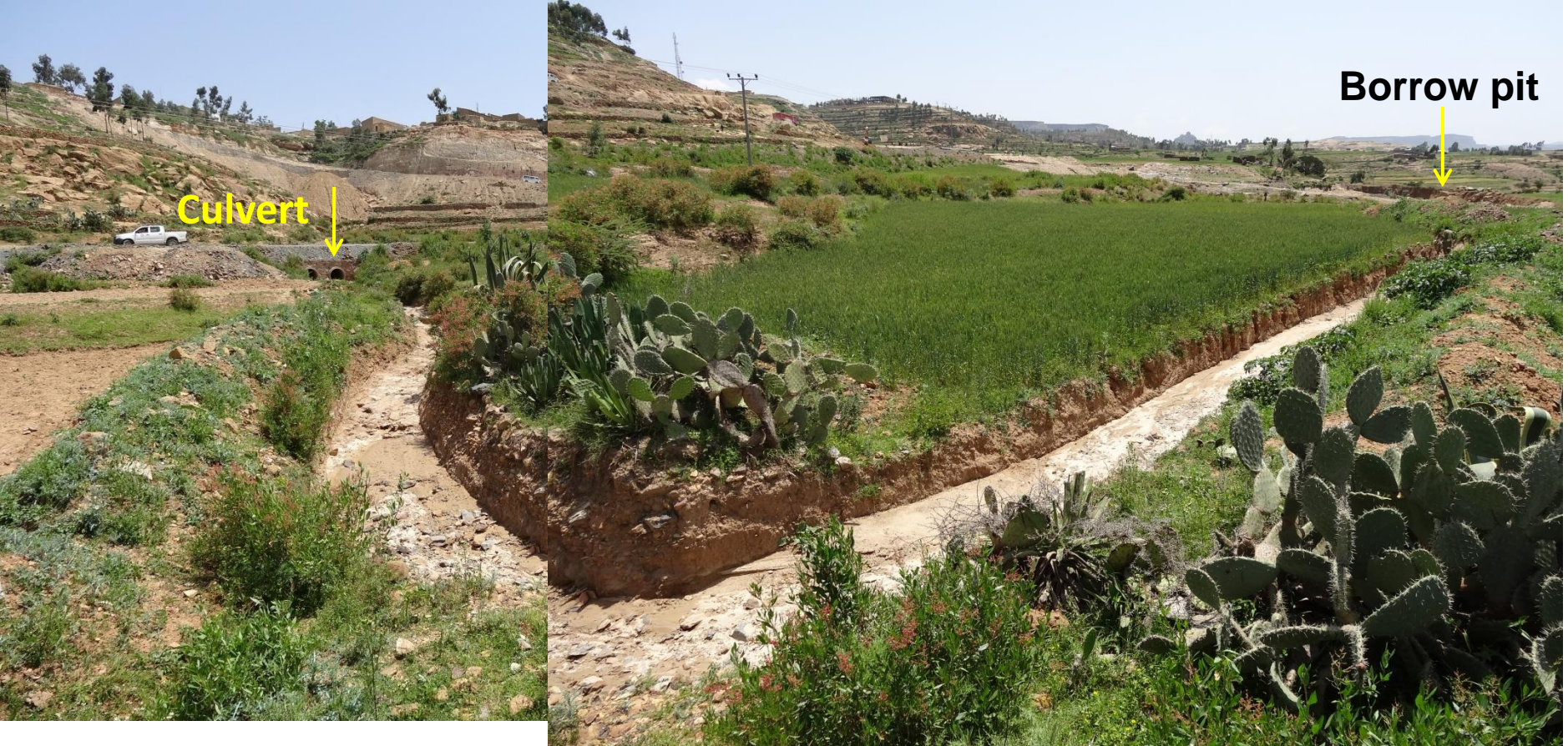
Plate 23. Panoramic view of channels constructed to divert water from culverts into a borrow pit shown in Plates 21, 22.
