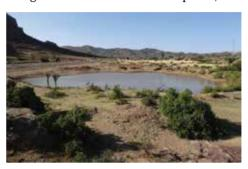
**Figure 2** Pond used to harvest runoff from culverts for livestock and groundwater recharge in Wukro area, Tigray, northern Ethiopia *Credit*: photo by Kifle Woldearegay, July 2013
