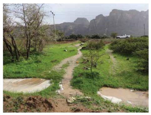
**Figure 4** Runoff from culverts being channelled to deep trenches in Hawzien area, Tigray, northern Ethiopia *Credit*: photo by Kifle Woldearegay, July 2013
