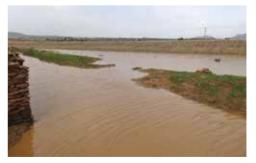
**Figure 1** Waterlogging behind a road embankment along the Freweign-Hawzien road, Northern Ethiopia *Credit*: photo by Kifle Woldearegay, July 2013
