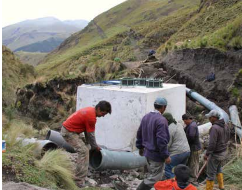
San Isidro residents repair an installation on the irrigation water pipeline during a day of communal labour. Photo: Tristan Partridge
