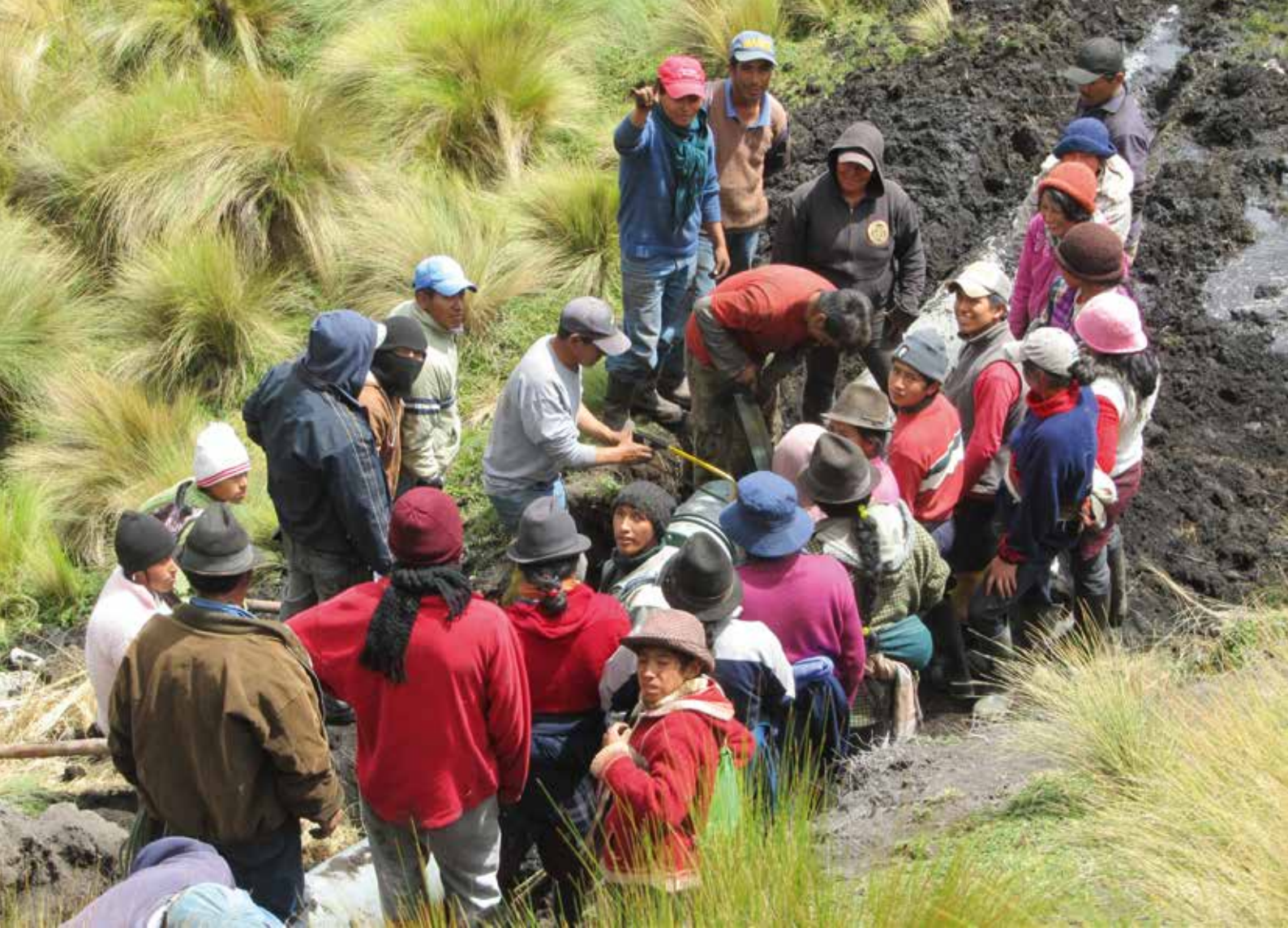
A day of communal labour in the San Isidro páramo repairing a section of the community's irrigation water pipeline. Photo: Tristan Partridge
