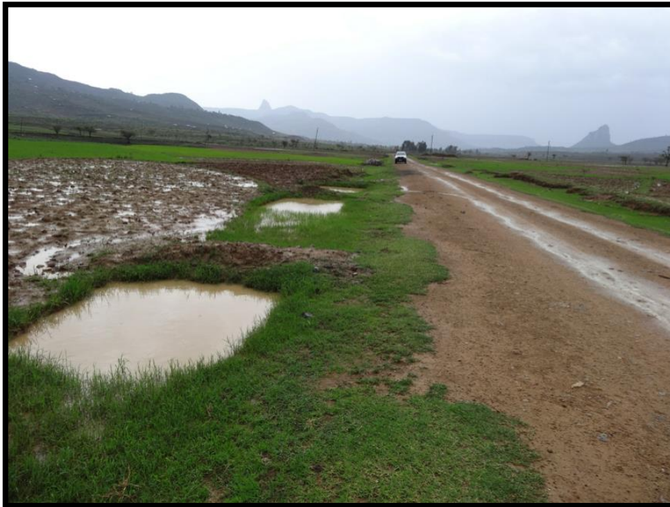
Figure 9: Road ponds are installed along the road to capture runoff and recharge groundwater (Roads for water, 2015).
