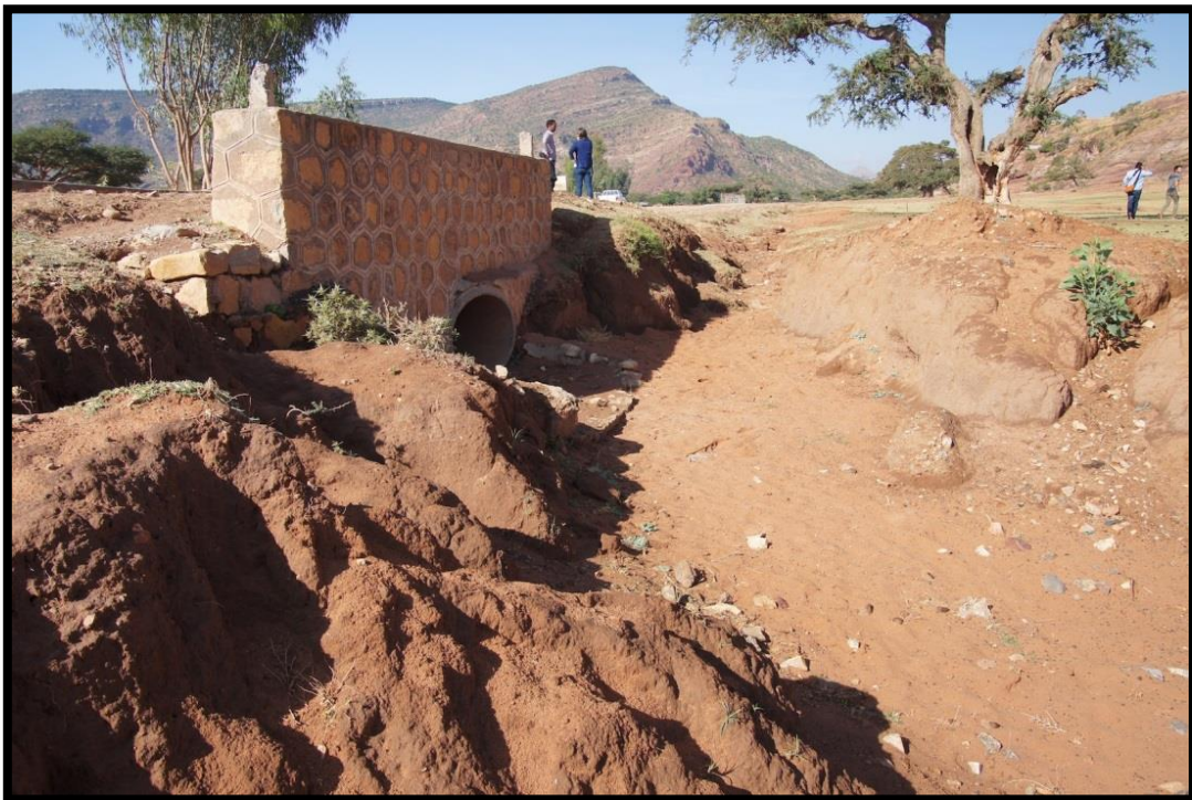
Figure 14: The photo shows a culvert surpassing a bridge along the surveyed route. The runoff from the culvert outlet and road side merge at this point and cause the development of a severe gully (Roads for water, 2015)
