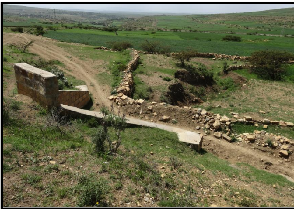
Figure 10: Culvert discharge is channelled and spread into farmlands, without adjustments the gully would most likely cause gully formation (Roads for water, 2015)
