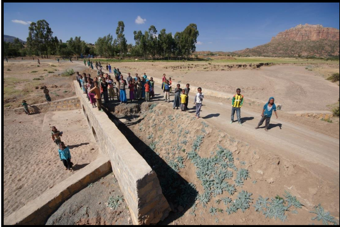
Figure 15: The photo shows a bridge that is completely ‘eaten’ by the high volumes of runoff from the road surface, the installation of an appropriate internal drainage system could have avoided this severe damage (Roads for water, 2015).
