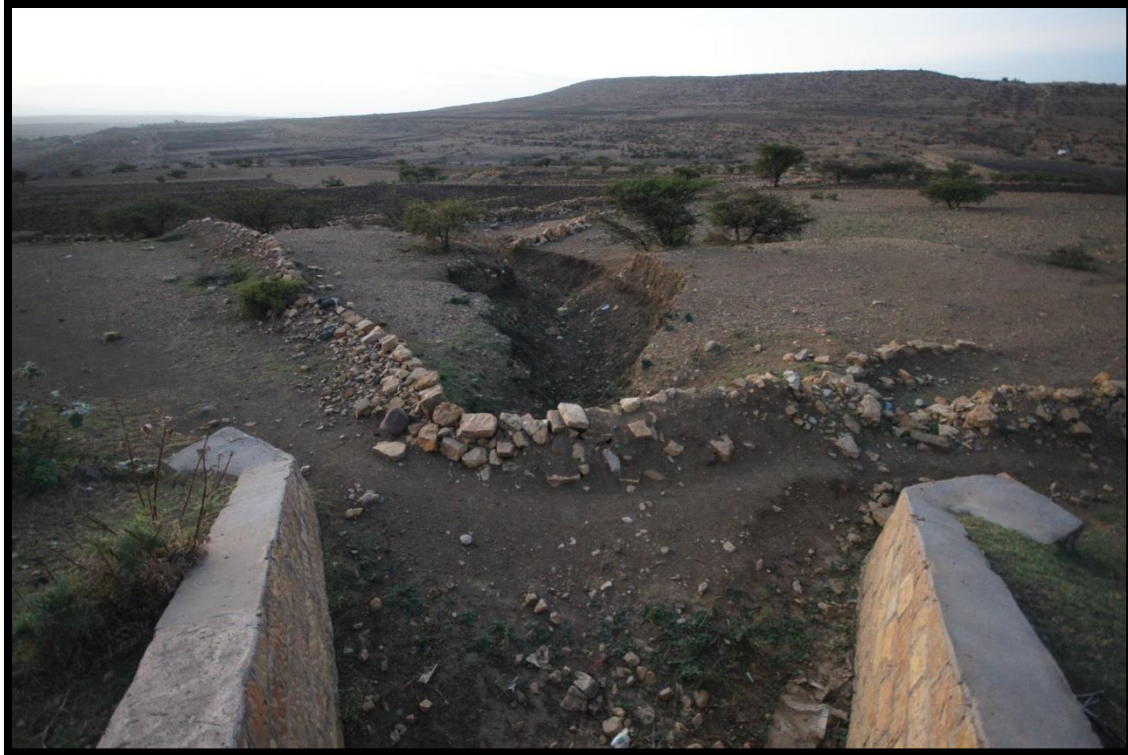
Figure 11: The photo shows the outlet from a cross-draining culvert. In the centre of the picture one can clearly see a previous developed gully. The culvert outlet is adjusted by stone bunds to reduce the runoff energy by diverting the flow in two parts, the gully can now be recovered (Roads for water, 2015).
