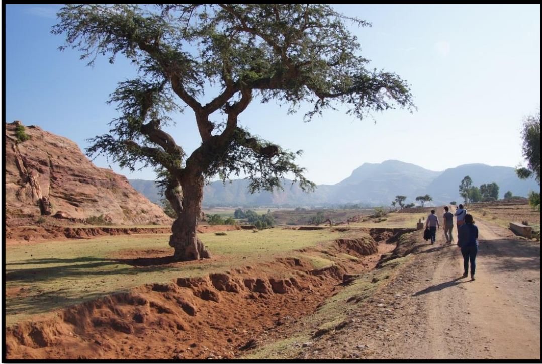
Figure 13: The photo shows part of the surveyed route. The road side is characterised by a large gully, developed due to a too concentrated flow caused by an insufficient drainage design (Roads for water, 2015).
