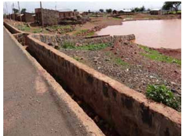
But roadside drainage can be diverted to groundwater percolation ponds (Ethiopia)
