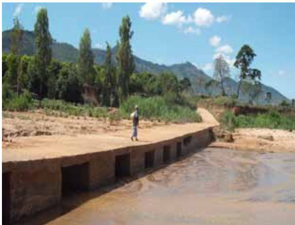
Road crossing retaining water in river bed in Kenya
