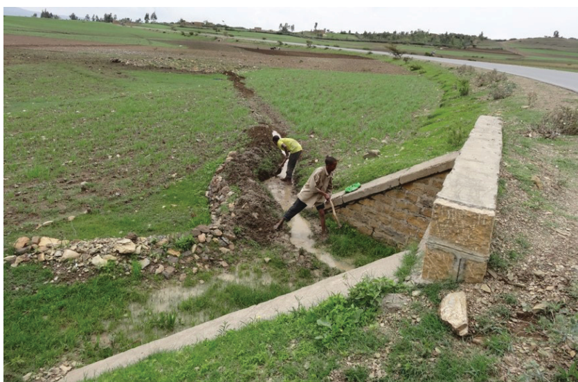
Communities digging a trench to divert water from the road to farmland
