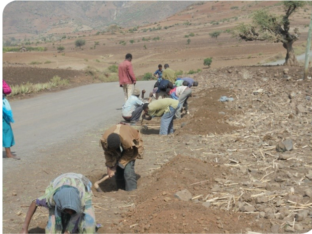
Communities building roadside trenches during the mass mobilization campaign
