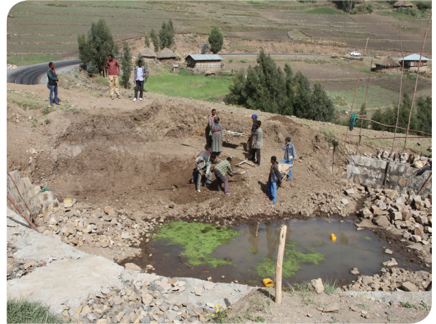
Building a pond to protect the road
