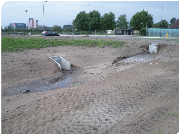
Swallow for groundwater recharge in the Netherlands
