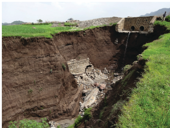
Gully created by excessive run-off from culvert Photo credit: Mekelle University
