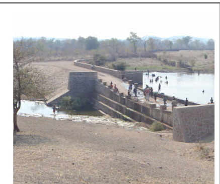
(2) Road crossing doubling up as dam/sand dam in Mozambique
