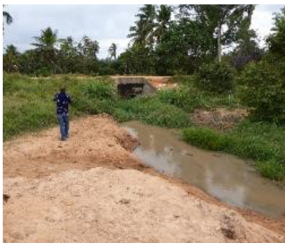
(3) Large deposits of washed away road material
