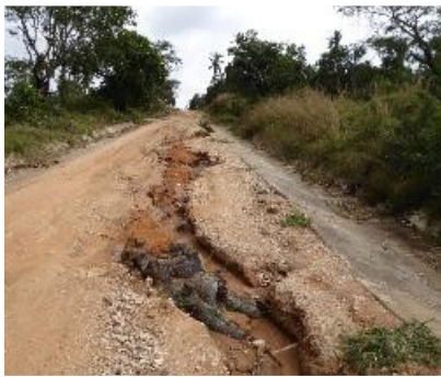
(1) Massive gullying on red sand road slope
