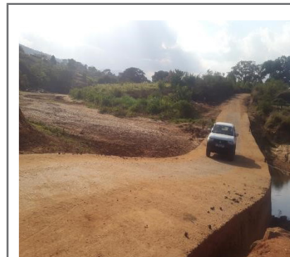
(1) Non-vented drift doubling up as sand dam in Kenya
