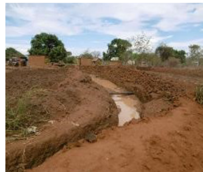
(4) Improved practice in Kenya – farm road trench filled with water
