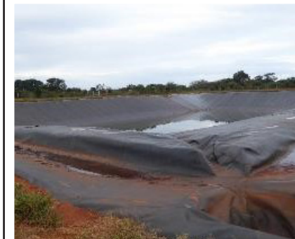
(4) Mavanza upgraded borrow pit – with geomembrane lining and fencing – intensely used
