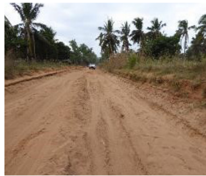
(2) Road lowered 90 centimeter due to wash out
