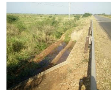
(2) Bridge on N1 – bridge sill level determining moisture levels in sugercane growing area
