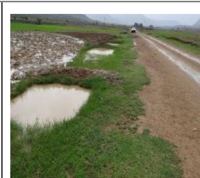
(4) Road side infiltration trenches – all pictures from Ethiopia – note that the distance to the road is too small
