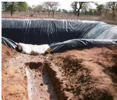
(3) Improved practice in Kenya – trench and pond
