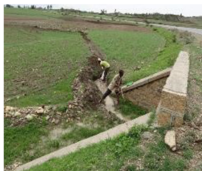
(2) Flood water spreader from culverts
