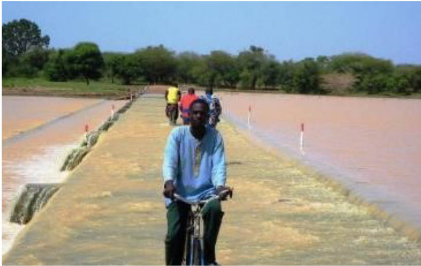
(1) Road cum flood water spreading weir in Niger
