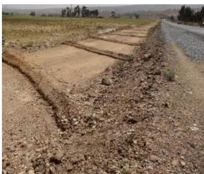
(1) Flood water spreader from paved road surface
