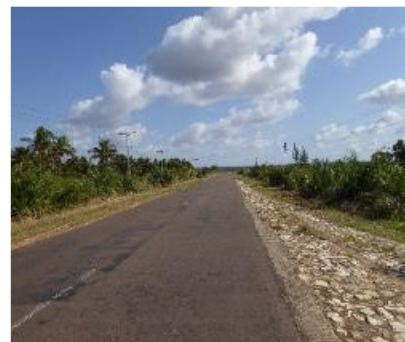
(4) Good practice of low embankment road in Lindella – with armoured overflow area complete with flood velocity reducing trees along the overflow area
