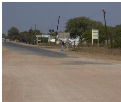
(3) During floods the same road was overtopped and wash away – with extensive damage
