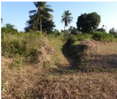
(1) Short road trench – standard practice now
