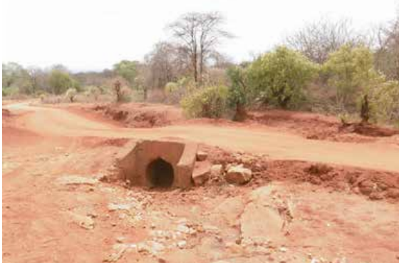
Figure 9: Side culvert scoured out, road trajectory re-allocated on the right side. Down: New cross-culvert on new road is causing erosion and gully-formation in side drain.
