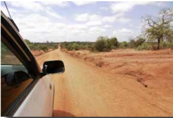
Figure 7: Road stretch, showing sedimentation and erosion on the side
