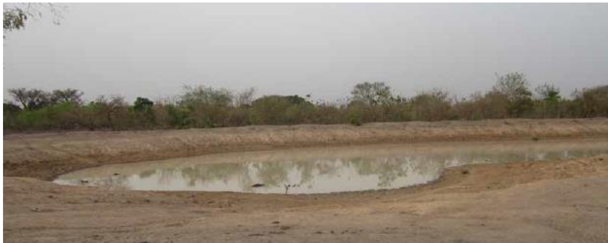
Figure 3: A borrow pit filled with seepage from high shallow groundwater in South Sudan. Photo: MetaMeta.
