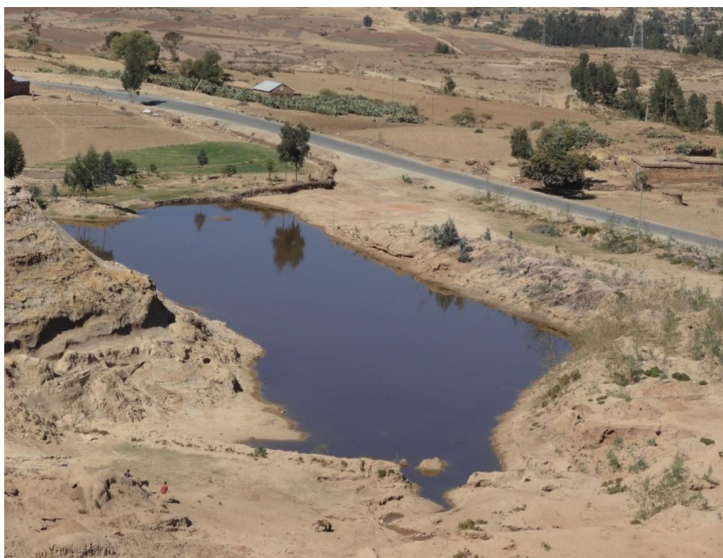
Figure 1: Road-side water harvesting in a borrow pit in Ethiopia. Photo: MetaMeta.
