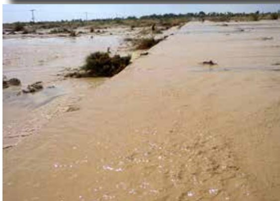
Figure 4: Road crossing at Kot Kaisrani (Pakistan), the upstream riverbed is stabilized with the construction of a drift
