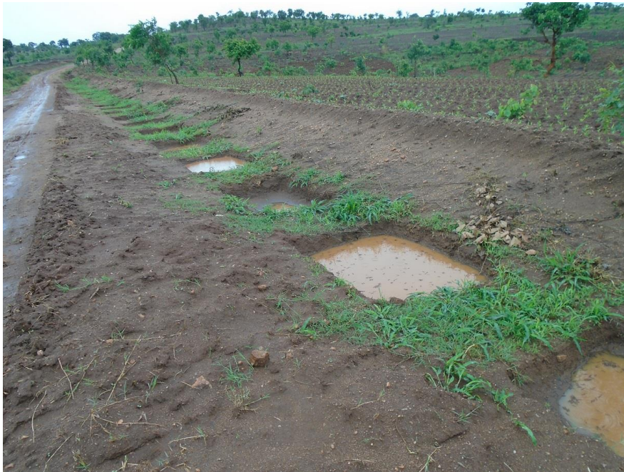
Roadside Pits (Chiwamba EPA)
