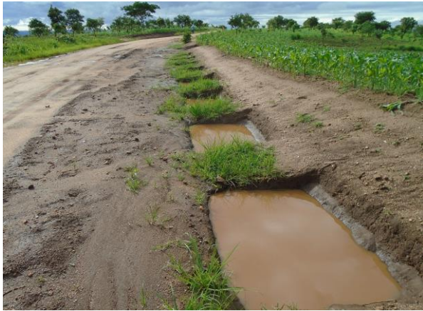
Road side pits
