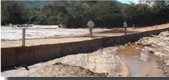
Figure 6: Non-vented drift crossing a river in Kenya
