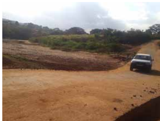
Figure 2: Example of non-vented drift, acting as sand dam to retain the sand upstream, Makueni, Kenya.
