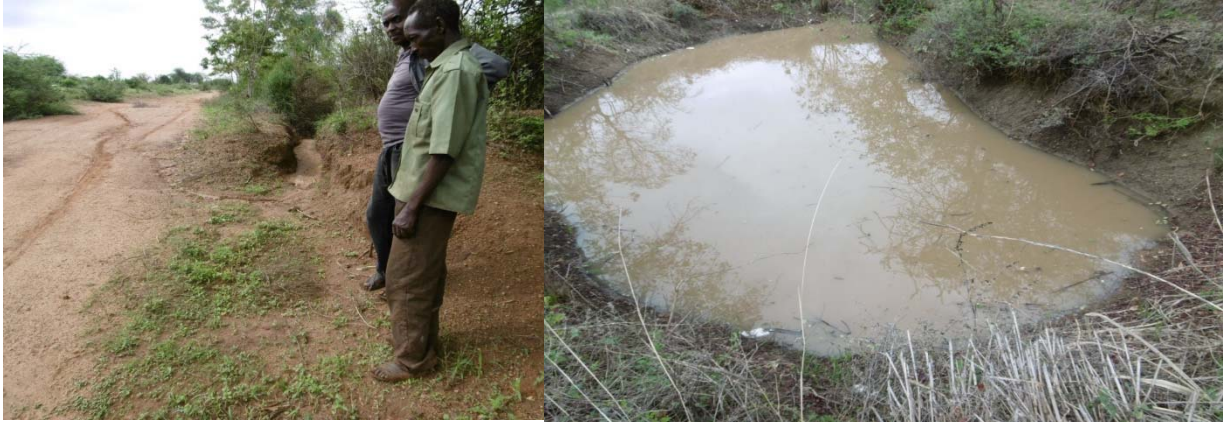
Figure 1 Munywoki Musya is harvesting road runoff which is stored in a pond within the farm
