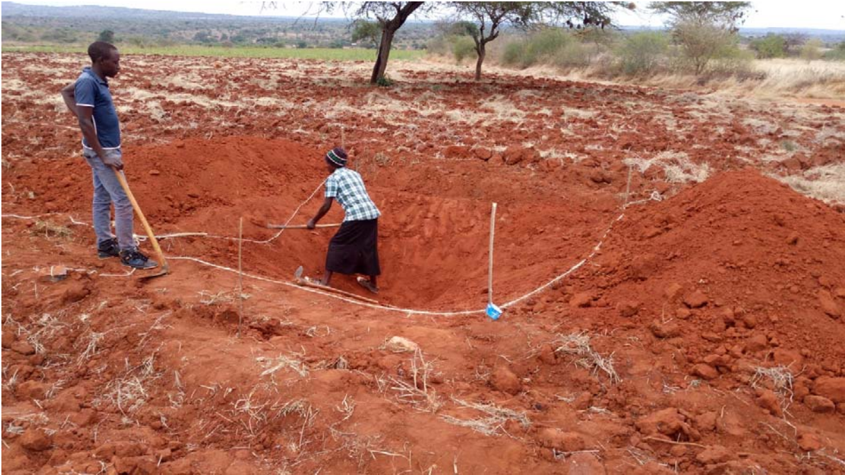
Figure 2: Casuals during the pond construction
