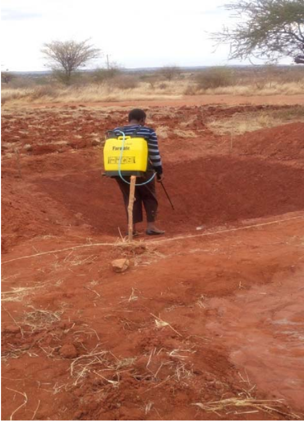
Figure 4: Spraying Terrasil on the compacted layers.
