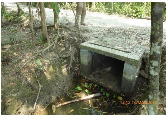
Figure 9. Box culvert with slot for gate
