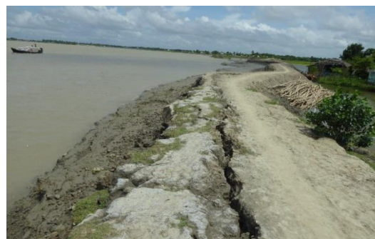
Figure 12. Too narrow and low embankment. High erosion and breaching. Ward 3, Kamarkhola.
