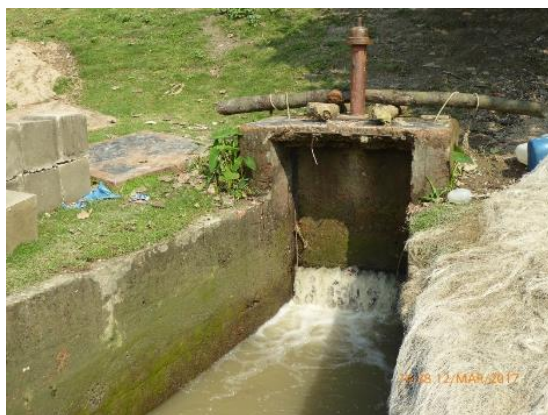
Figure 4. Defective sluice gate: this gate can neither retain water when it is needed (water losses) nor block water from entering when it is not needed (flooding). Figure 5. Drainage congestion around a house. This photo was taken in March 2017 during the dry season, 2-3 days after a rain event
