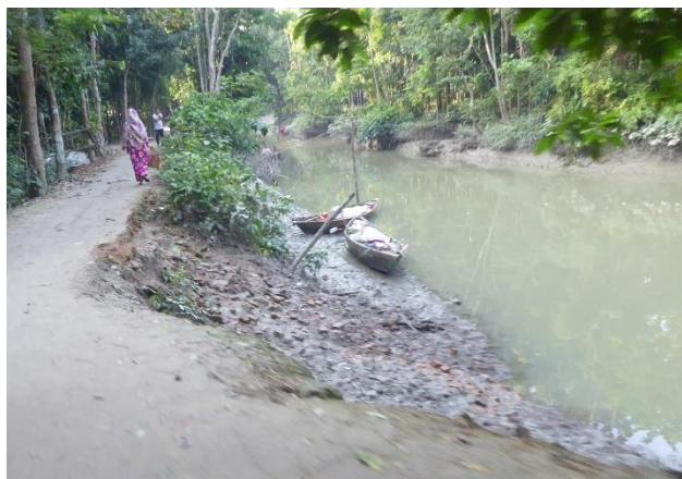
Figure 8. Silted khal and eroded side slope
