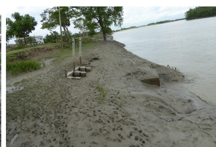
Figure 5. Silted sluices
