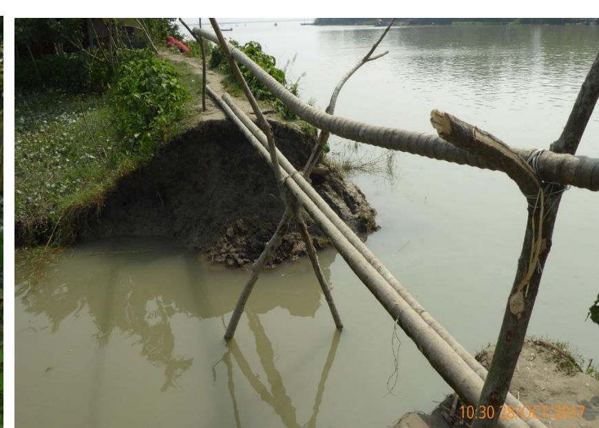
Figure 7. Embankment breaching
