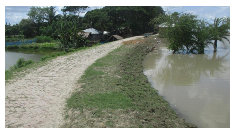
Figure 10. Road embankment as flood defense
