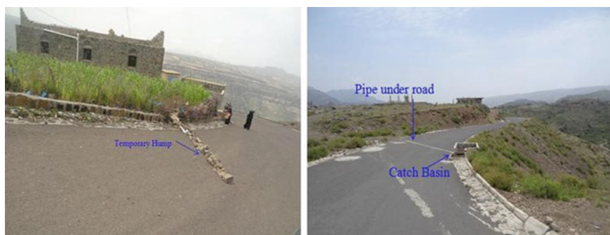
Fig. 15 Temporary hump diverting water from road surface to farmland and catch basin collecting road runoff and transporting it under the road. Photograph Mohammed Abdullah Al-Abyadh
