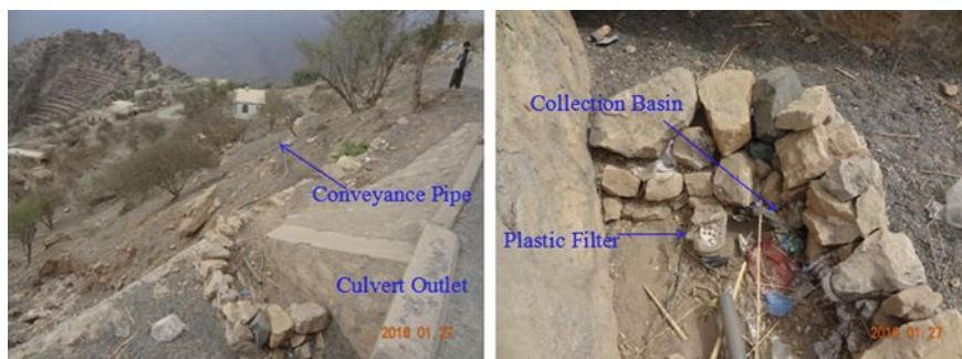
Fig. 14 Water from a culvert is gathered in a collection basin and transported through a polyethylene pipe. Photograph Mohammed Abdullah Al-Abyadh
