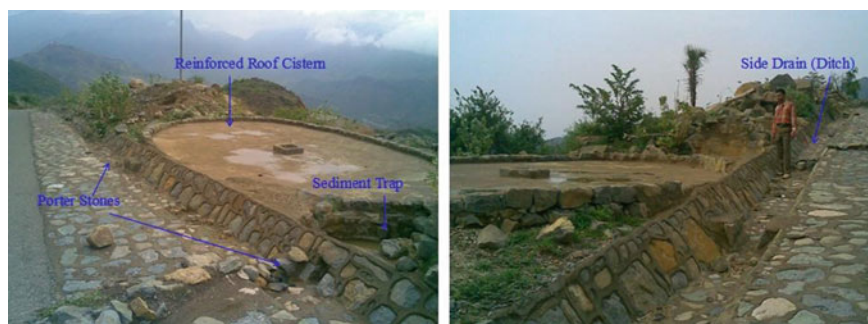
Fig. 13 Roofed roadside cisterns collecting road runoff in Yemen. Photograph Mohammed Abdullah Al-Abyadh
