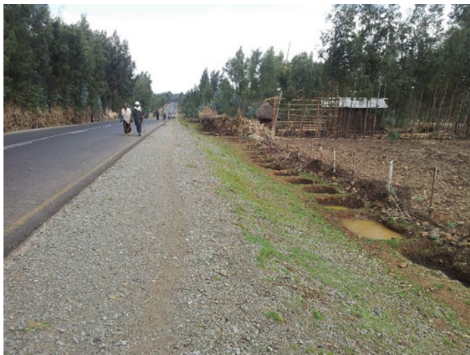
Fig. 3 Infiltration trenches along an asphalt road in Amhara Region, Ethiopia. Photograph Marta Agujetas
