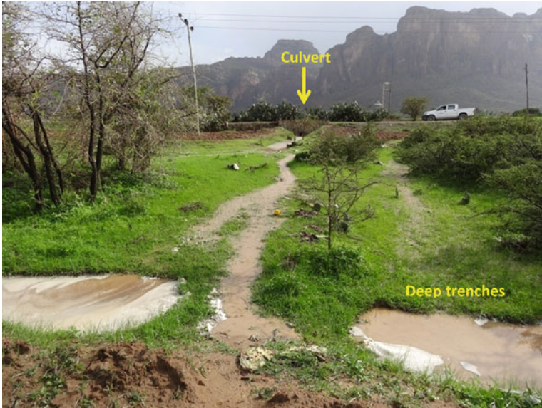
Fig. 6 Water from a culvert is channelled into a deep trenches in Megab area, Tigray, Ethiopia. Hand-dug well downstream of these trenches is used for monitoring. Photograph MetaMeta
