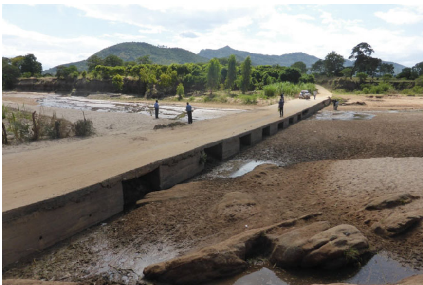
Fig. 5 Road crossing doubling up as a sand dam in Makueni, Kenya. Photograph MetaMeta
