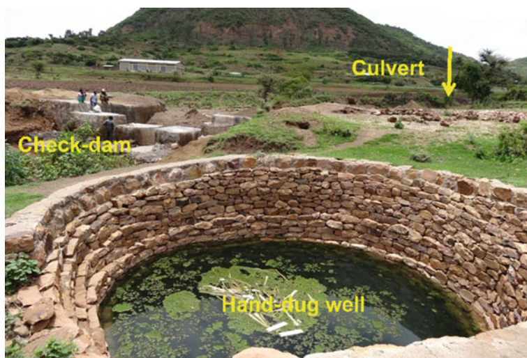
Fig. 10 Channelling water from a culvert into a check dam is enhancing groundwater in Seleklele area, Tigray, Ethiopia. Photograph Kifle Woldearegay
