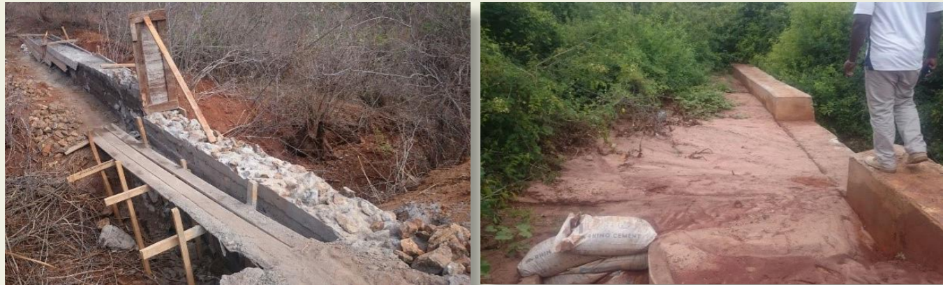
Figure 8 Check-dam before (left) and after (right), installation combined with a pond
