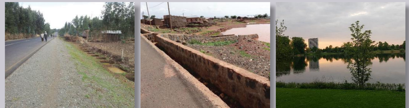
Figure 7: example of road water harvesting in urban setting, creating infiltration pits and water (recharge) reservoirs
