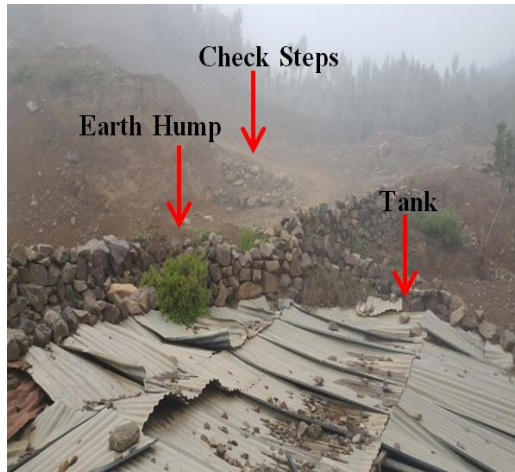
Figure 25 Right: Earth check steps to divert the surface runoff to the tank by earth hump, Left: Open water harvesting tank and an earth hump
