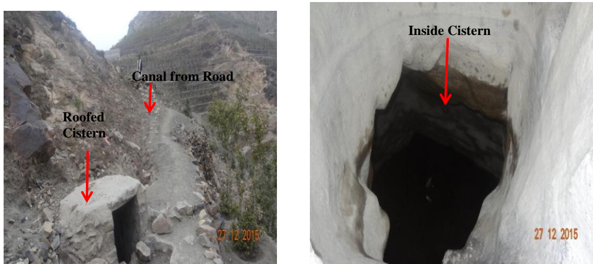
Figure 23 Roofed Dug Cistern near the main road
