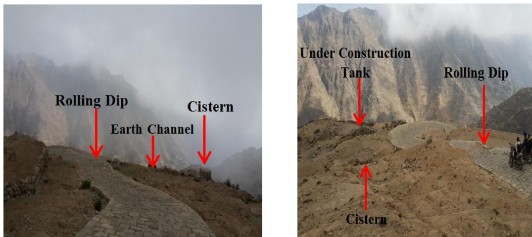
Figure 28 Stone paved rolling dip to divert rainwater to the tanks
