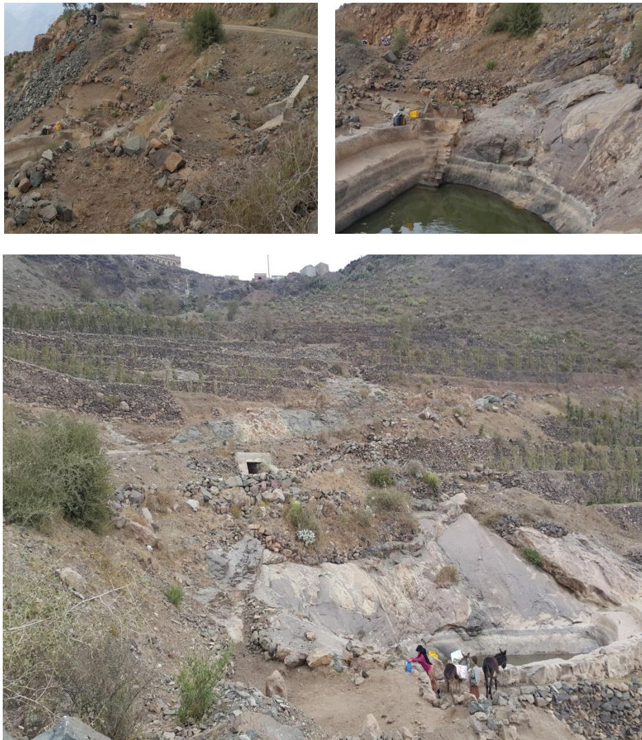
Figure 75 Water harvesting pond from culvert outlet
