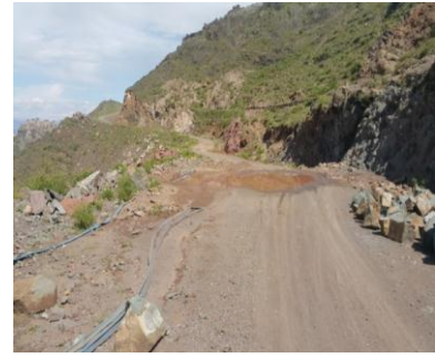
Figure 74 The earth hump which constructed by the farmer to intercept the road runoff and the right water channel but as the gradient is up-sloped the farmer use a plastic tube to convey the intercepted water to the tank by using in situ pump. It also shows the hill and part of the strip catchments.
