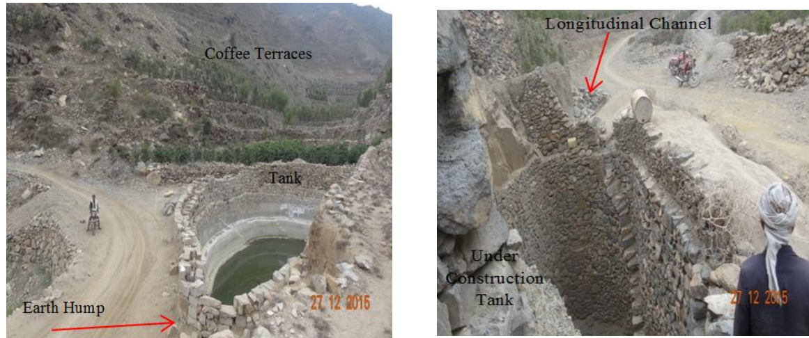
Figure 20 Left: Open water harvesting tank near coffee terraces, Right: Under construction water harvesting tanks
