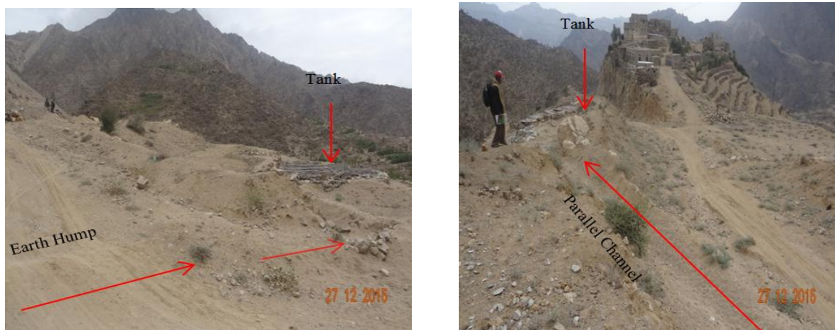
Figure 21 Left: shrubs roofed water harvesting tank the farmer use an earth hump to divert the water from the road surface. Right: old corrugated roofed tank the farmer use parallel side ditch to divert the water from the road.
