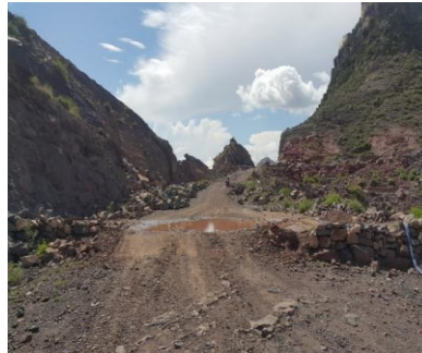
Figure 74 The earth hump which constructed by the farmer to intercept the road runoff and the right water channel but as the gradient is up-sloped the farmer use a plastic tube to convey the intercepted water to the tank by using in situ pump. It also shows the hill and part of the strip catchments.
