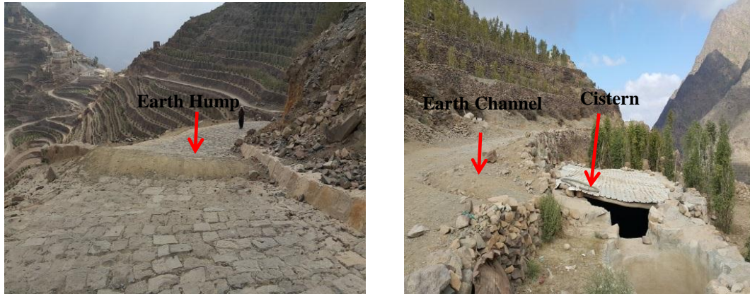
Figure 27 Rainwater diverting earthen humps and earthen channel
