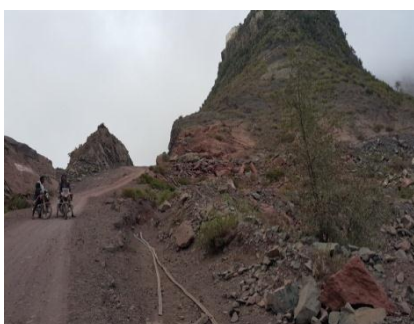
Figure 74 The earth hump which constructed by the farmer to intercept the road runoff and the right water channel but as the gradient is up-sloped the farmer use a plastic tube to convey the intercepted water to the tank by using in situ pump. It also shows the hill and part of the strip catchments.
