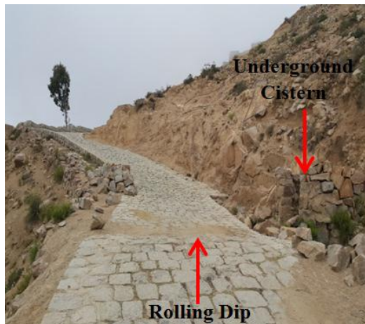
Figure 26 Underground cistern at the inner edge of the stone paved road
