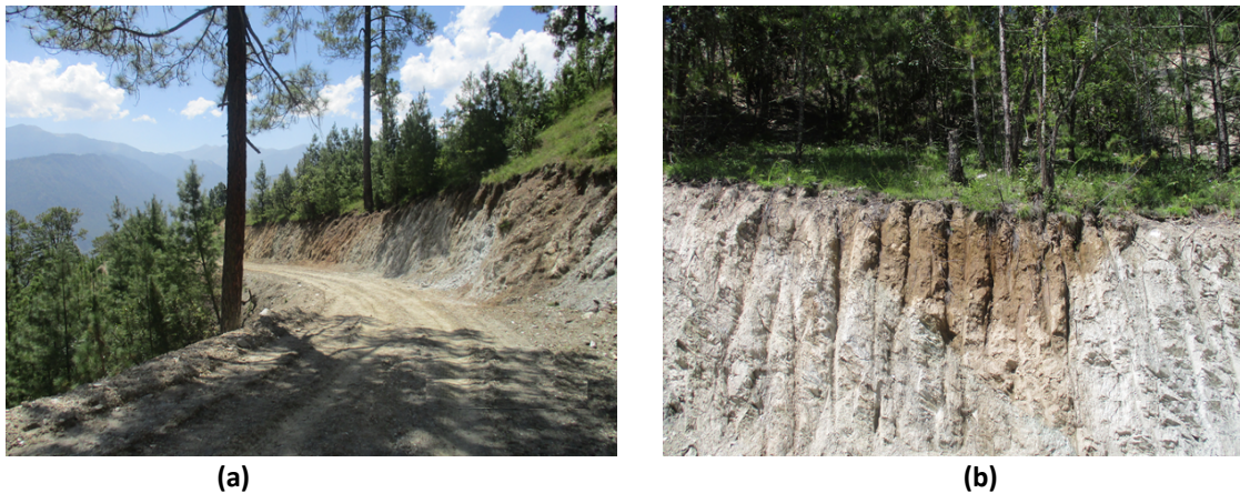
Figure 2: (a) Increased air-surface exposure of hill slope and (b) Interrupted subsurface flow due to road openings (photo taken at Dumkot area of MHLR road)
