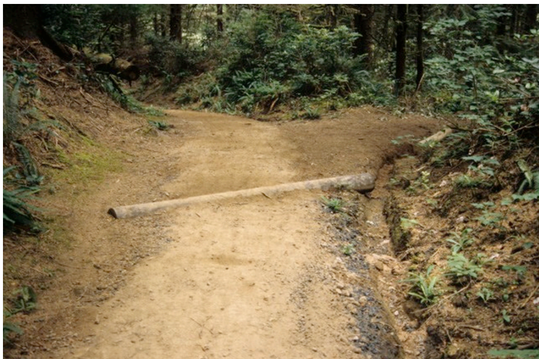
Figure 14: Water bar in the place (source: United States Forest Service, 2017)
