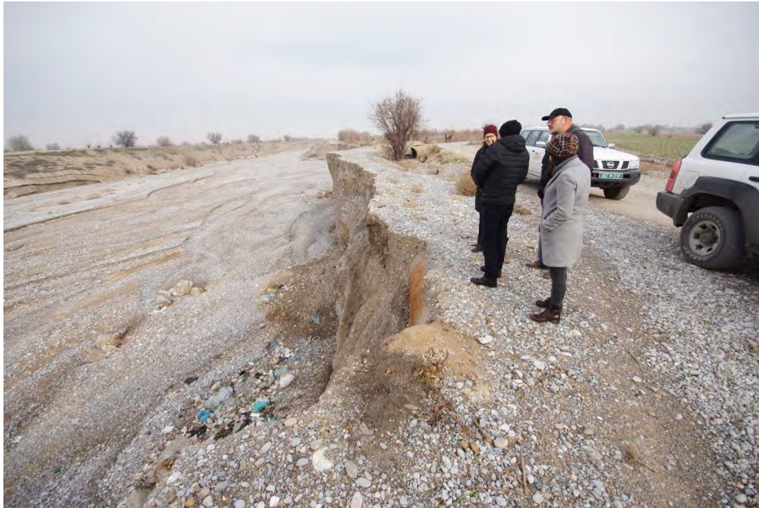
Plate 3: the external bend of the river, 8m above the canal. Observe the buried (rusty) pipeline linking two portions of the irrigation canal at the feet of the team, on right bank. On the left bank (the inside of the bend), some concrete slabs remain (Source: Author)..
