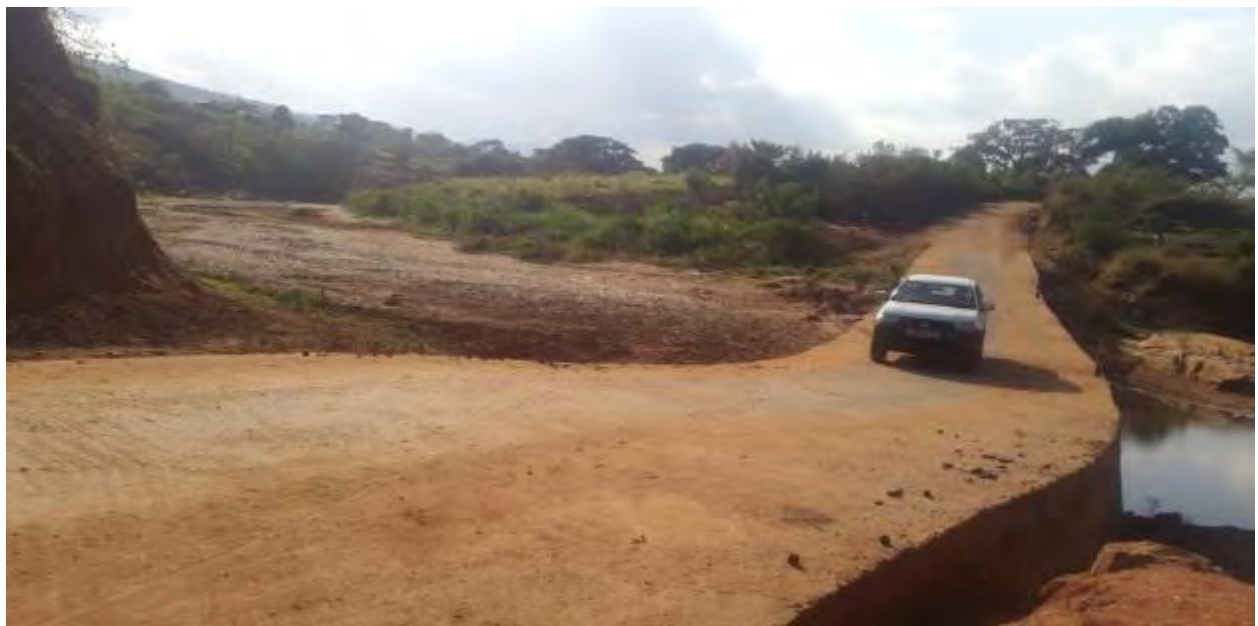
Plate 15: Non-vented drift stabilizing dry river and acting as sand dam (Source: Author)
