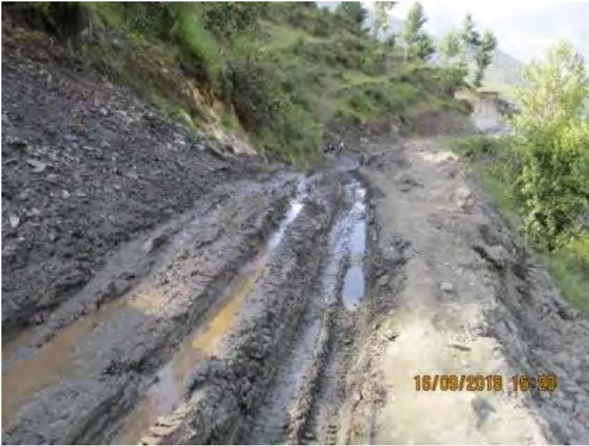
Plate 21: A seep opening up and damaging the road surface (Source: Author)
