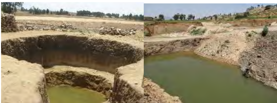
Plate 23: Collecting road water for groundwater recharge: Recharge well (Ethiopia) and abandoned borrow pit (Mozambique) (Source: Author)
