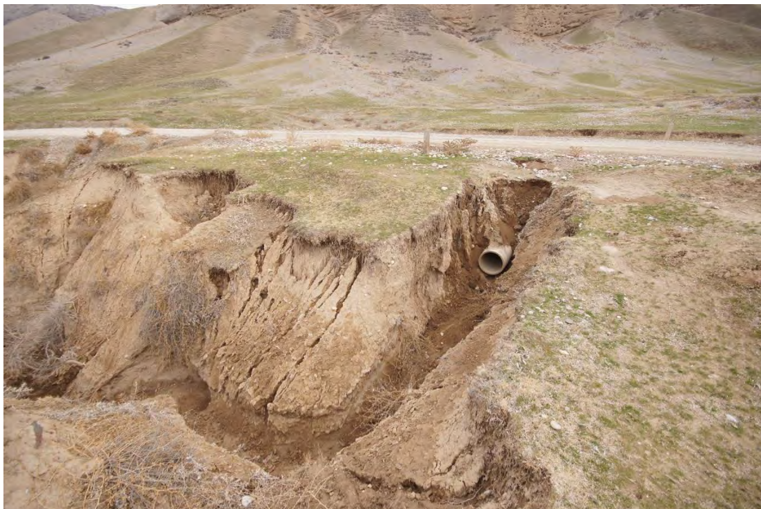
Plate 6. Gullies triggered by the culvert (Source: Author)
