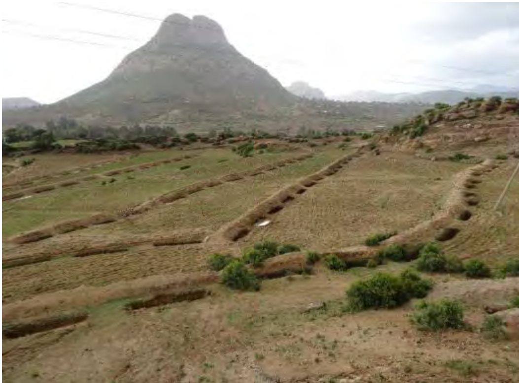
Plate 22: Series of roadside infiltration trenches with bund to intercept additional surface runoff, Tigray, Ethiopia (Source: Author)
