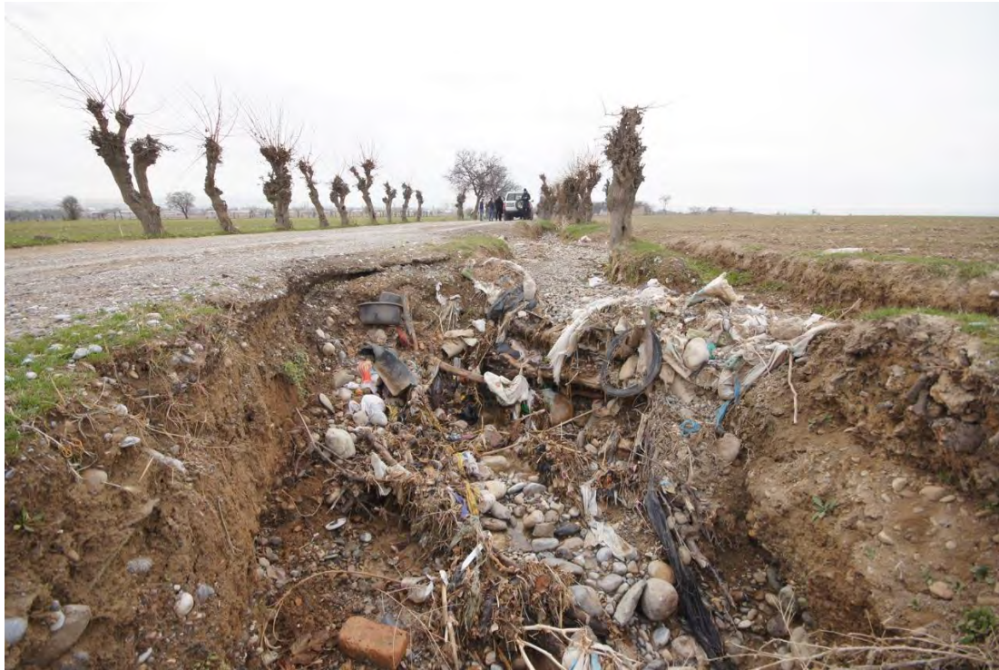
Plate 5. Erosion due to the runoff, threatening the road; garbage management issue (Source: Author)
