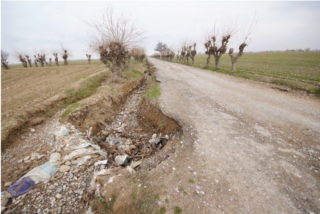
Plate 4. Erosion due to the runoff, threatening the stability of the road, and the fields (Source: Author)
