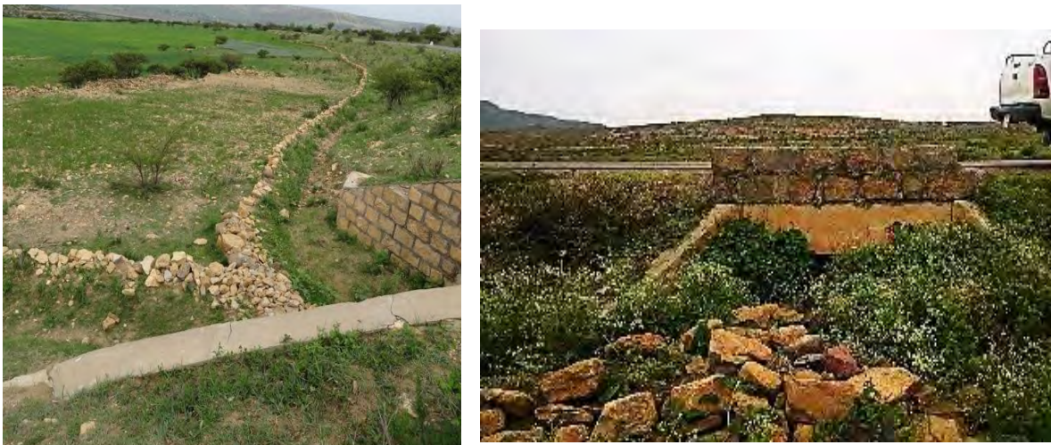
Plate 16: V-shaped diversion structure constructed from soil and stone to spread water from culvert, Ethiopia (Source: Author)
