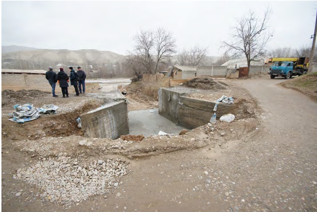
Plate 13: bridge under construction (Source: Author)
