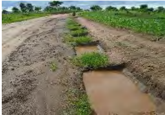
Plate 17: Infiltration trenches along roads: note these should be placed at distance for road safety and road integrity. the trench on the right (in Malawi) is too close to the road (Source: Author)
