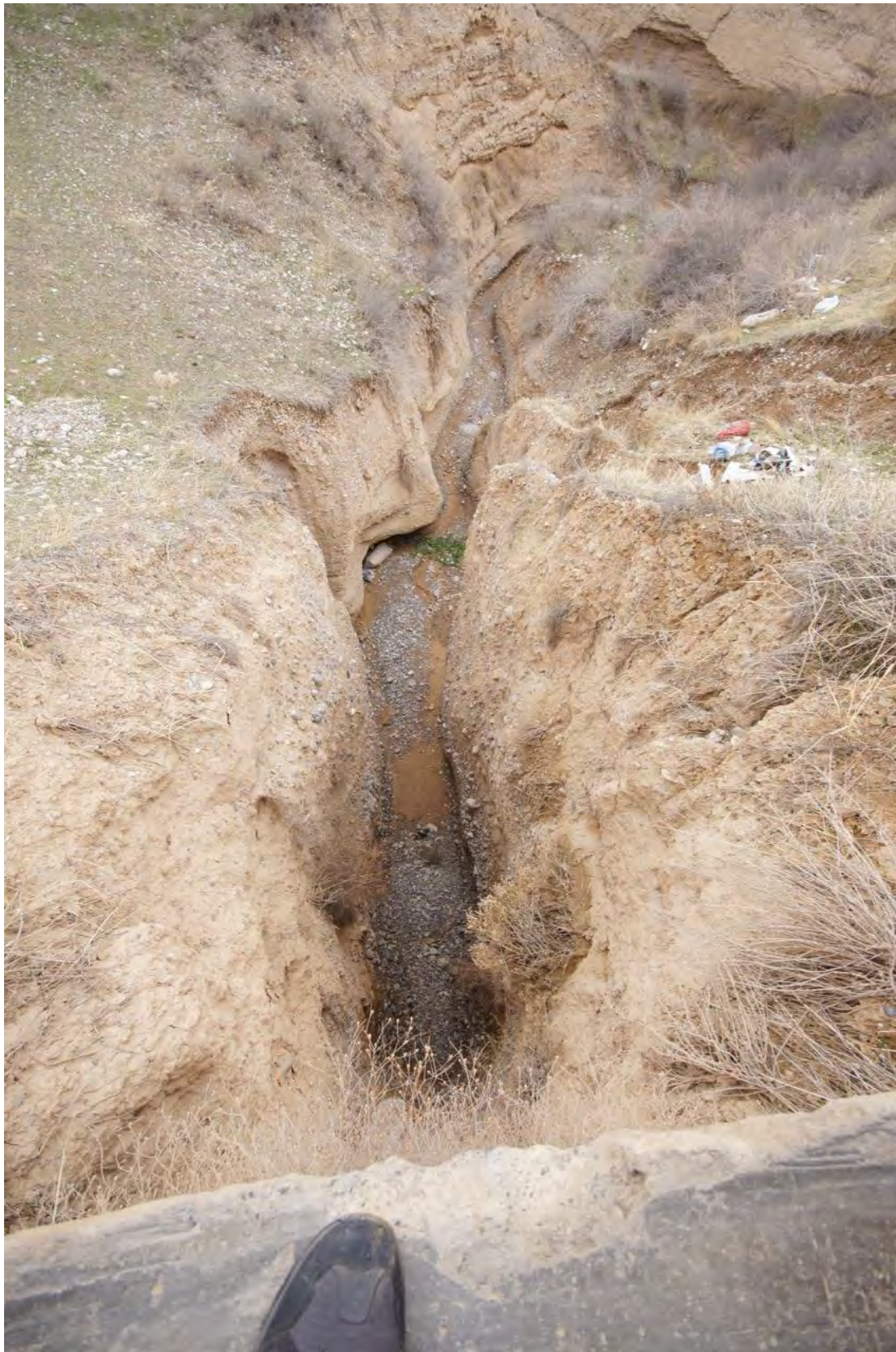
Plate 10. The erosion gully seen from inside the culvert (height: approximately 10m; Source: Author)
