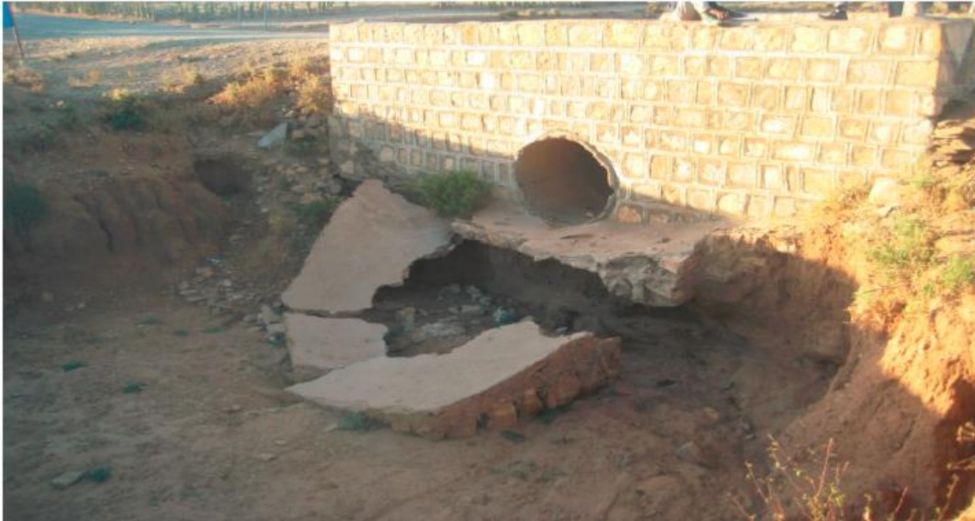
Fig. Example of gully formation downstream of a road along the Freweyni to Abreha-we-Atsibha road route
