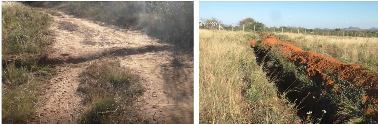
Figure 2: Road water harvesting intake and collection structures
