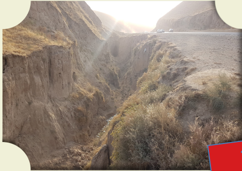
Erosion and sedimentation
