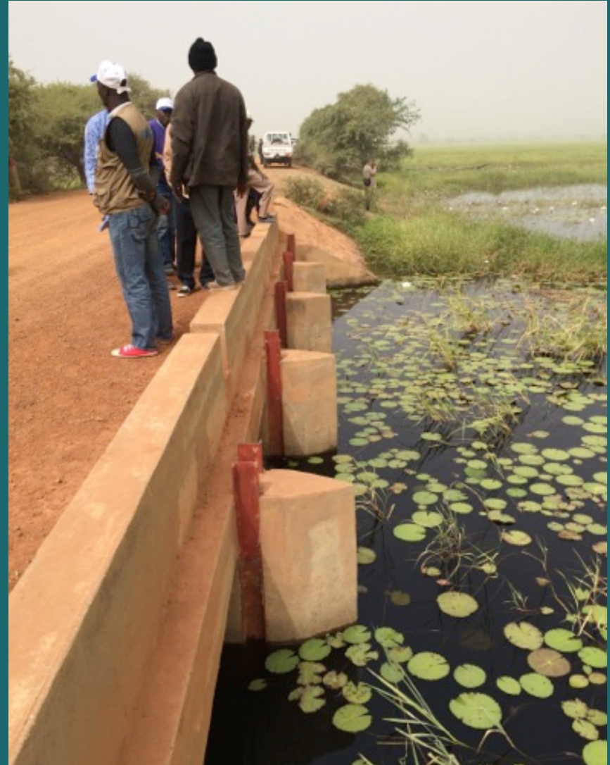
Road embankment creating storage reservoir
