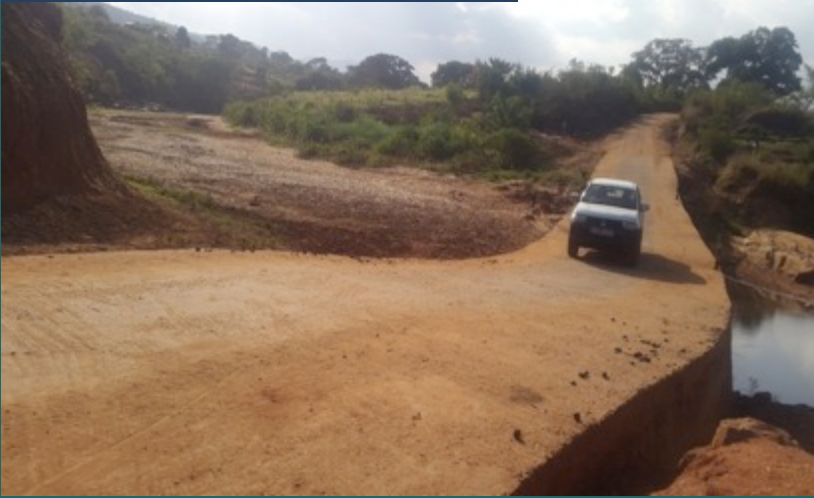
Retaining water with road drifts
