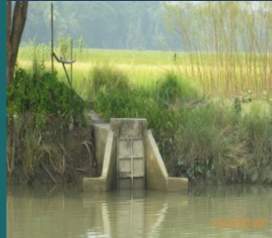
Gated culverts for water management
