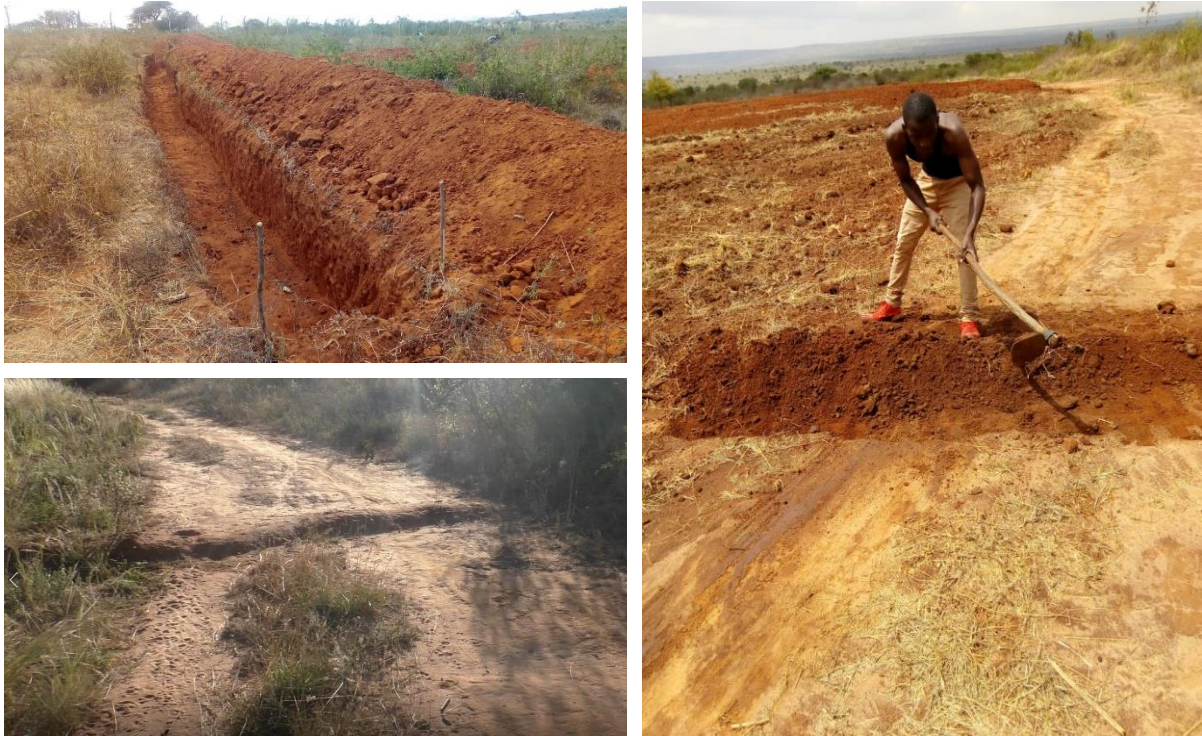
Figure 8 preparing road water harvesting diversion and collection structures in pasture land
