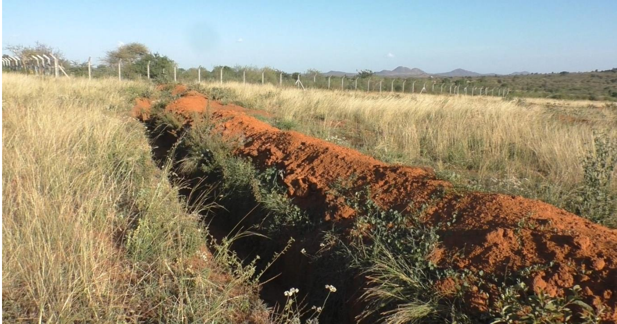
Figure 9 look-out of pastureland with trench slowing down water to infiltrate over longer time and prolong availability of soil moisture
