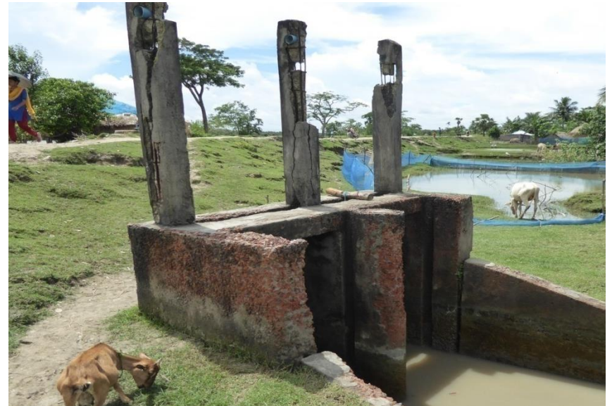
Can work but needs repair
