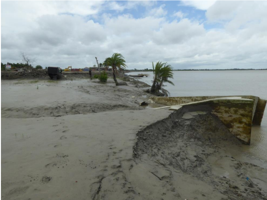
River erosion, tidal effect
