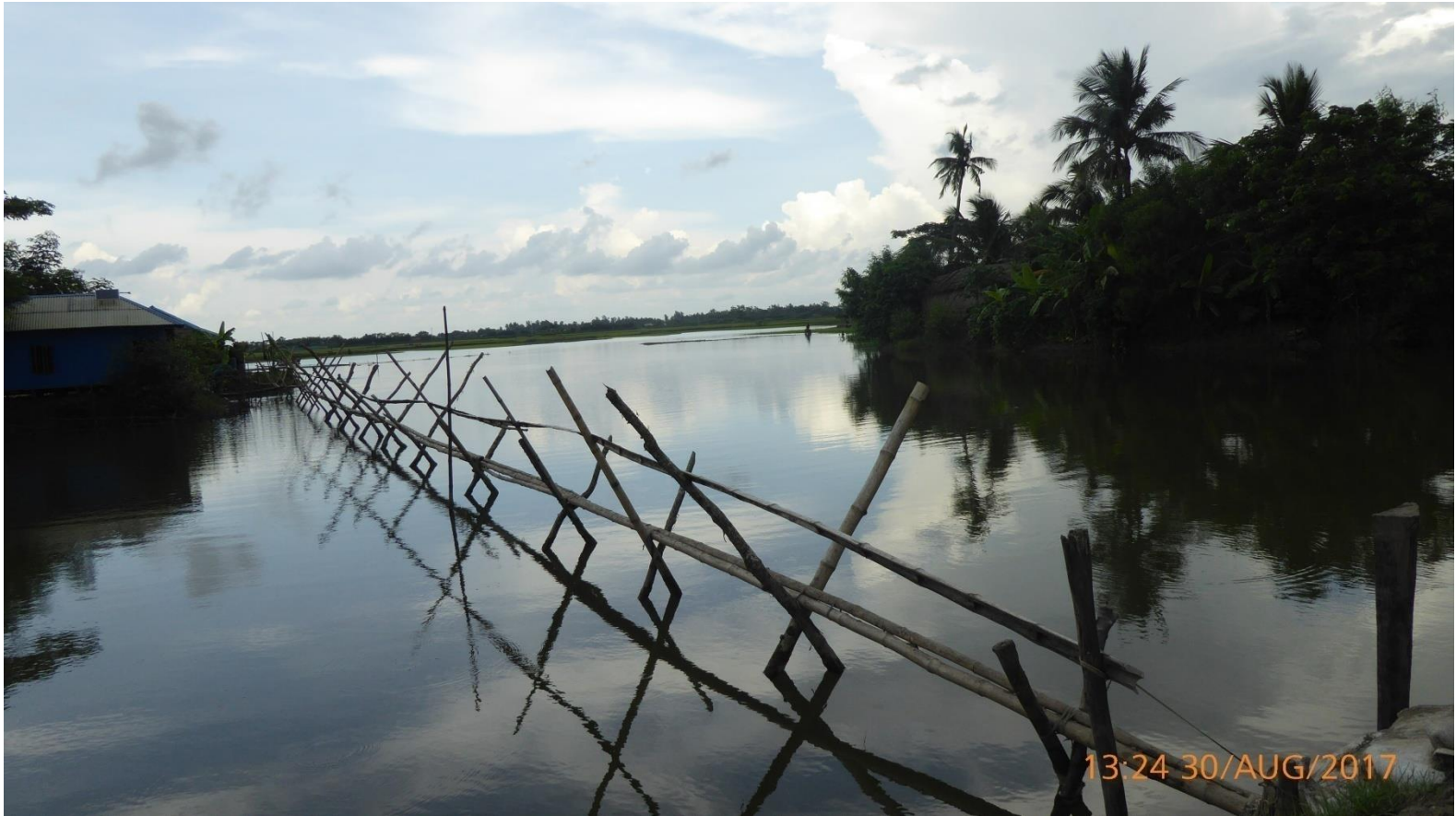
Water logging, no proper bridges/culverts
