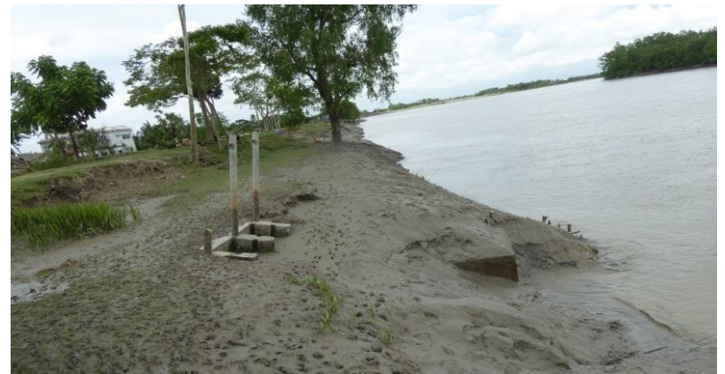
Silted sluice gates
