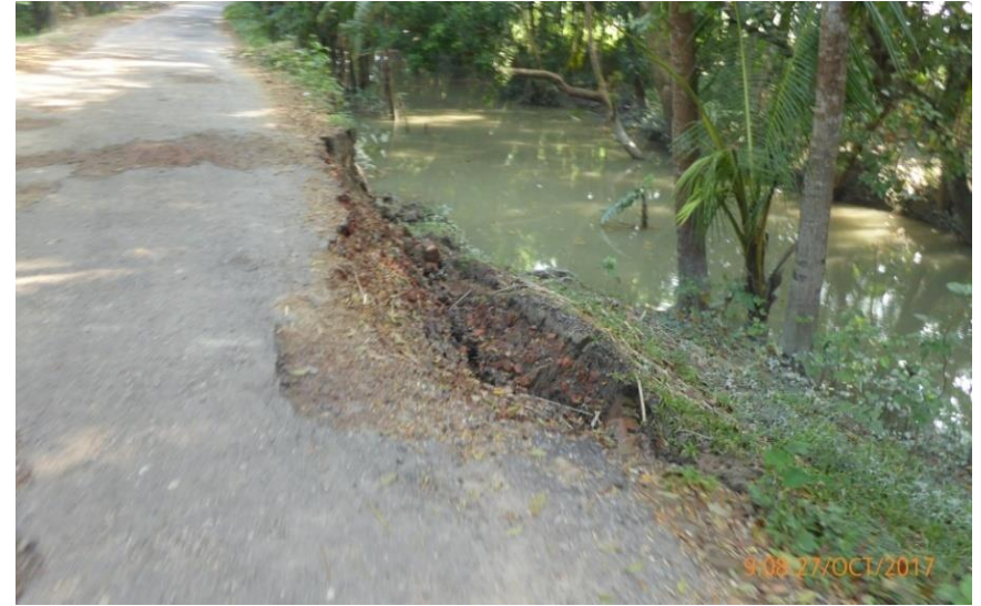
Broken sections of the road due to water erosion
