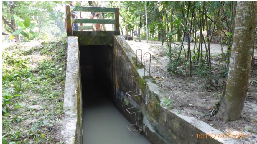
1V sluice gate
