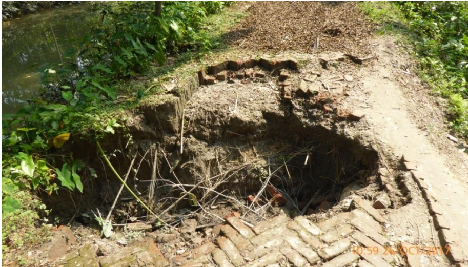
Road collapse, NO maintenance since 17 years
