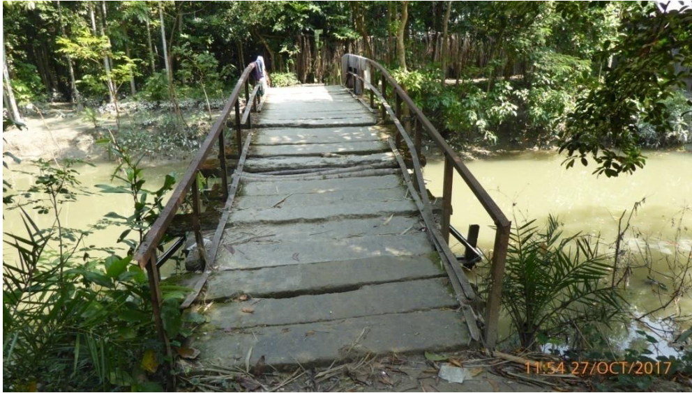
Old bridge needs repair/replacement
