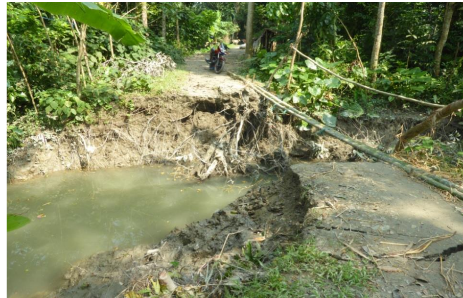
Road collapse, NO maintenance since 17 years
