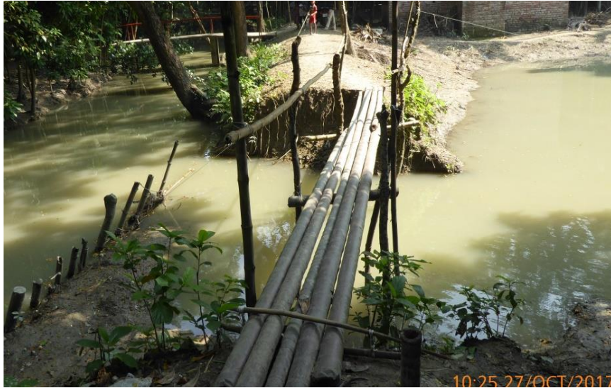
Broken sections of the road due to water erosion
