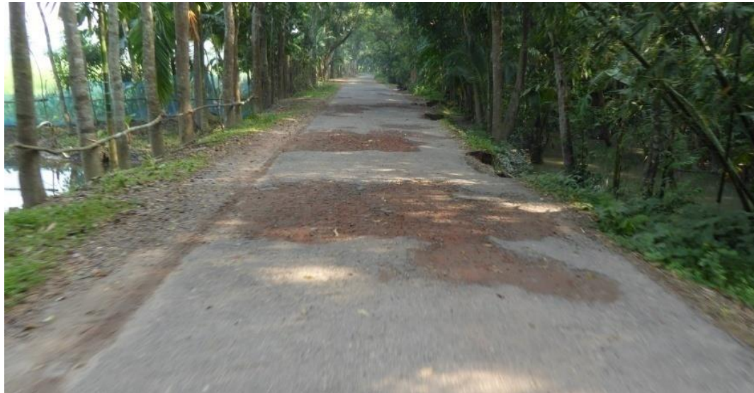
Broken sections of the road due to water erosion
