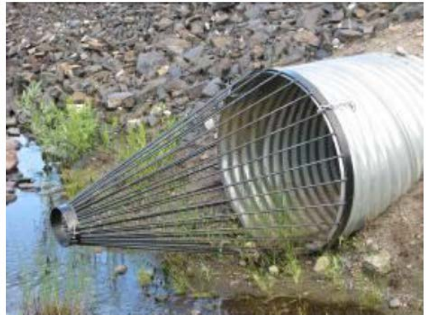
The Beaver Proof Add On (left) and the Beavercone (right) are examples of products that help prevent the damming or blockage of a culvert by beaver activity
