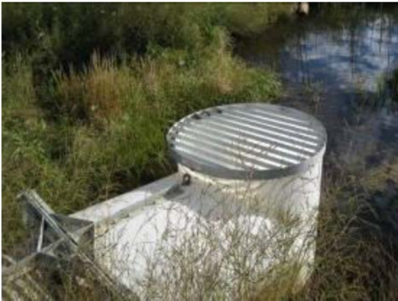
The Beaver Proof Add On (left) and the Beavercone (right) are examples of products that help prevent the damming or blockage of a culvert by beaver activity
