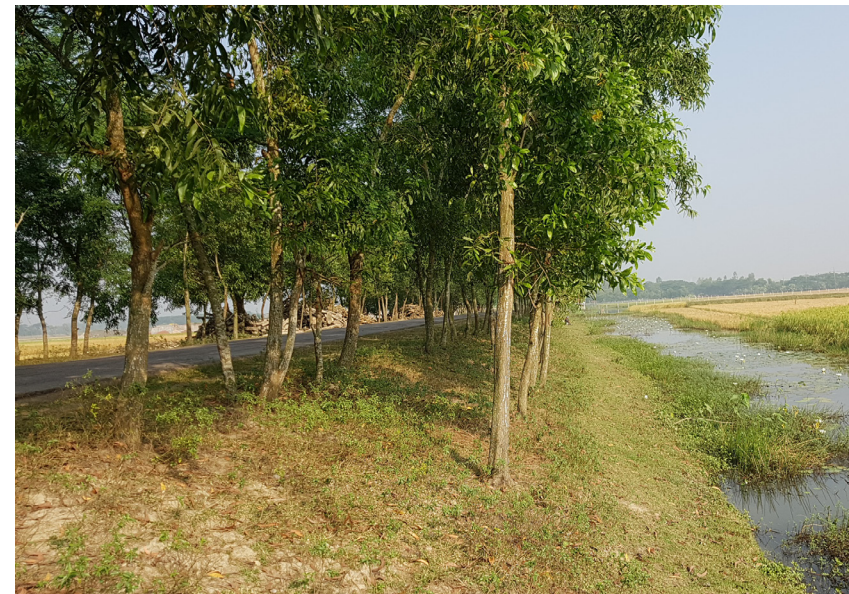
Borrow pits along the road for water management
