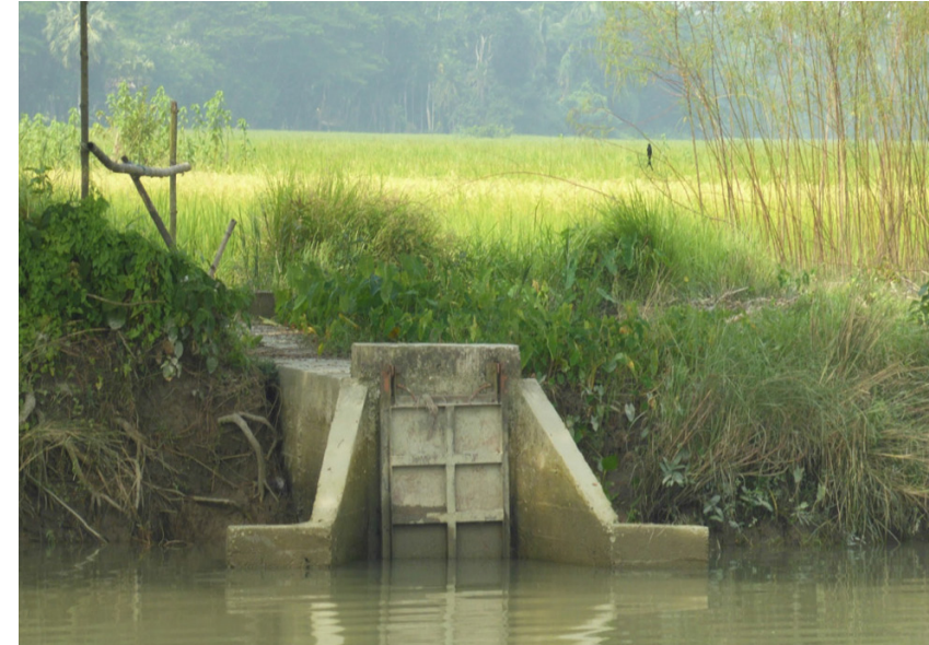
Managing water levels with gated cross drainage
