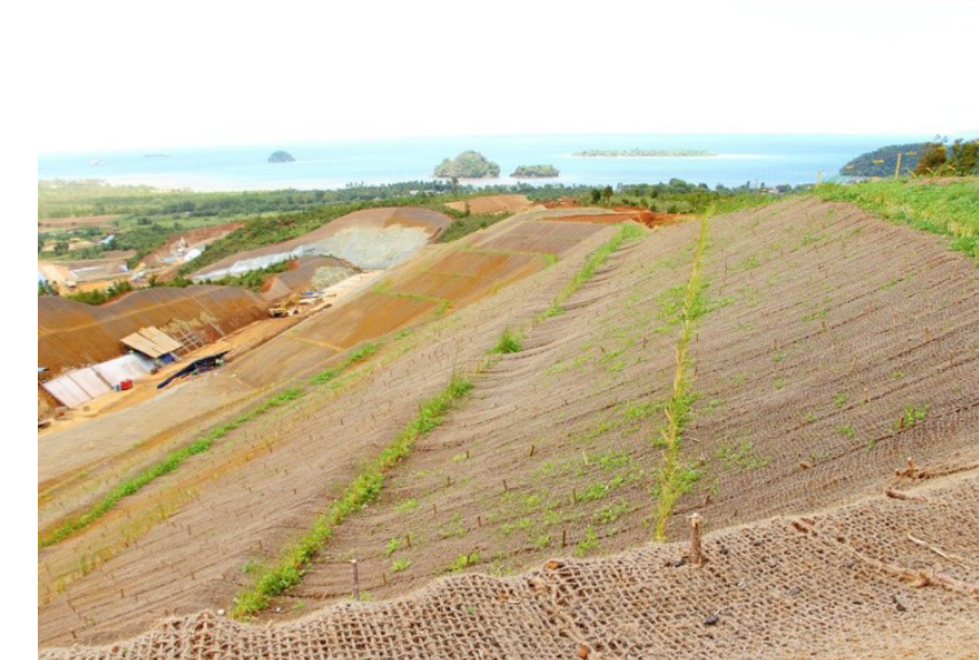
Use of turfing combined with jute netting for slope protection
