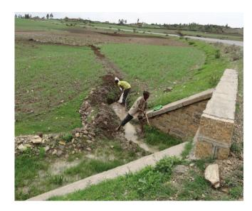
Flood water spreaders from road surface to enhance soil moisture and recharge groundwater
