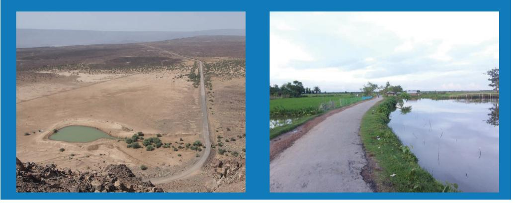
Water can be an important cause of damage to roads whereas in turn roads are a major cause for local flooding, compaction and erosion. These problems can be easily turned around into a potential. Roads can route water to storage ponds or recharge areas which help to retain water in dry riverbeds, and ensure systematic spreading of floodwater.
