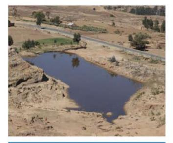
Water storage ponds to store water from road side drainages and culverts
