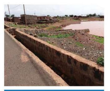
Roadside infiltration ponds for groundwater recharge
