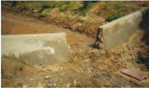
Stage 1. Spillway is 50 cm above the sand level.
