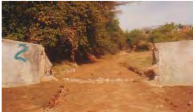
Stage 4. Flood has deposited sand to the new level of the spillway.
