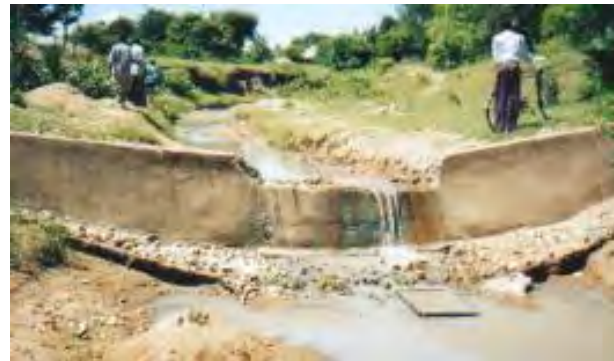
Stage 5. Spillway is raised to 50 cm above new sand level.
