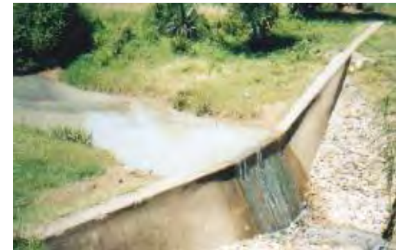
Stage 6. This procedure is repeated until the spillway is fully closed.
