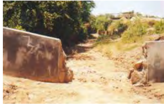
Stage 2. Flood has brought sand to the level of the spillway.
