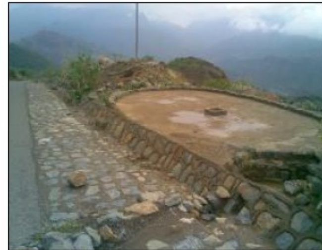
Water Harvesting cisterns from road side drains, Yemen (from Abyad 2013).
