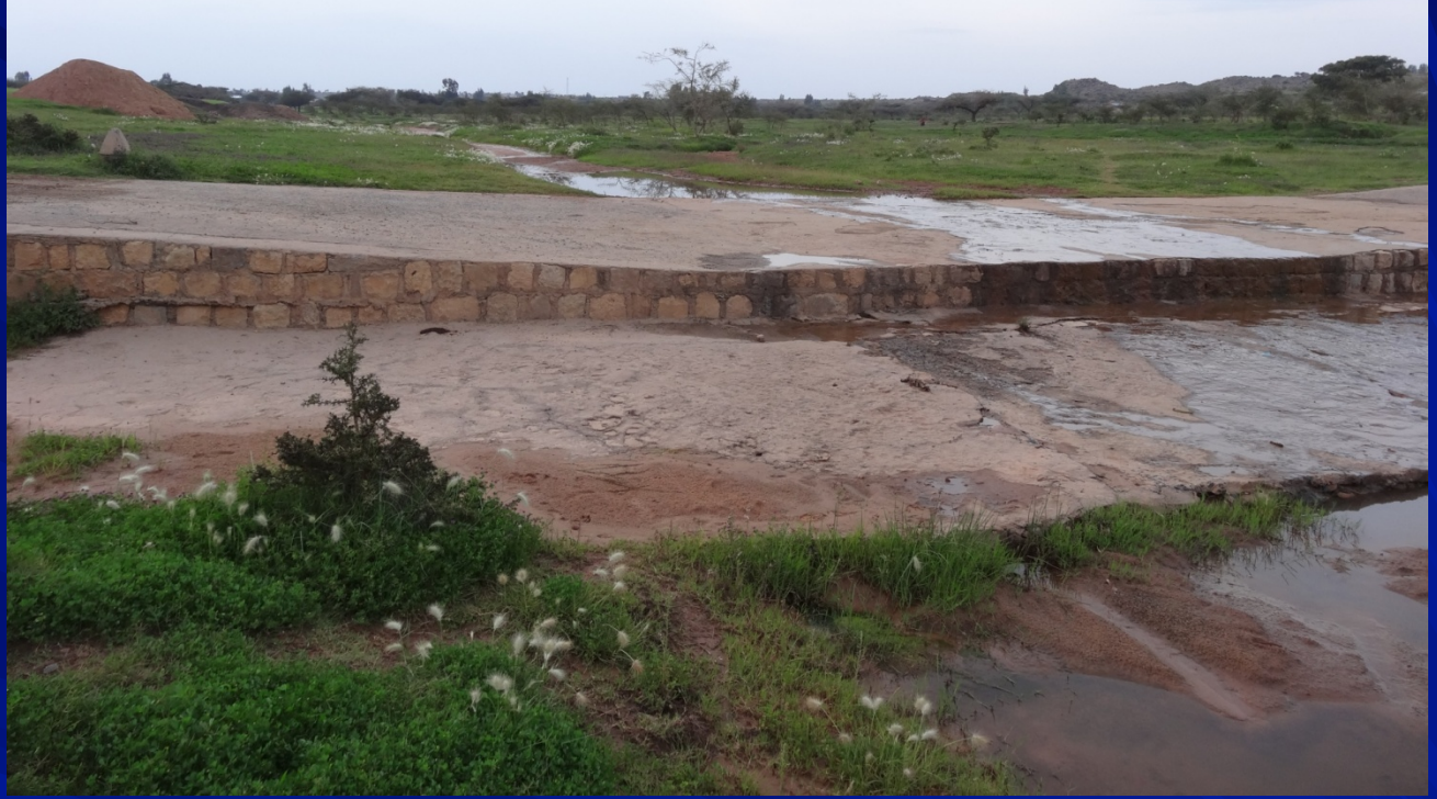
Irish Bridge (Photo: Sept. 01, 2013)
