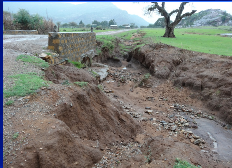
Gully erosion: water from culvert.
