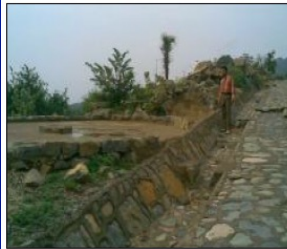
Water Harvesting cisterns from road side drains, Yemen (from Abyad 2013).
