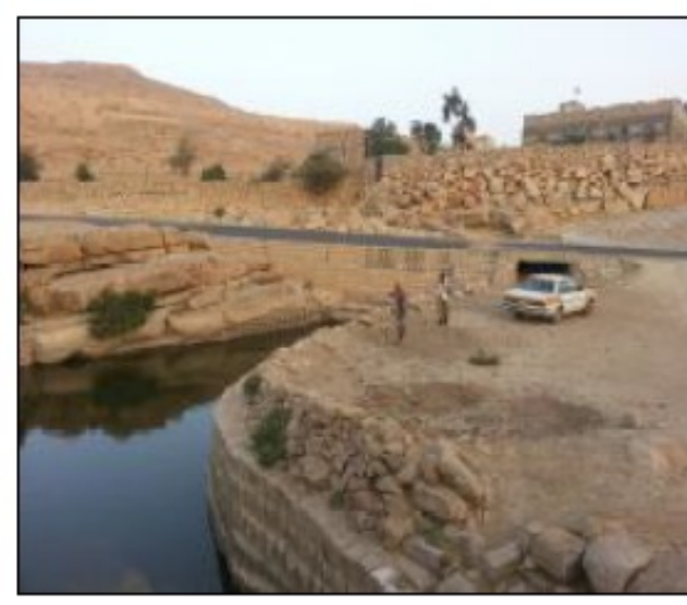
Water harvesting of road runoff, side drains and culvert into small pond, Yemen (REF Abyad 2013)
