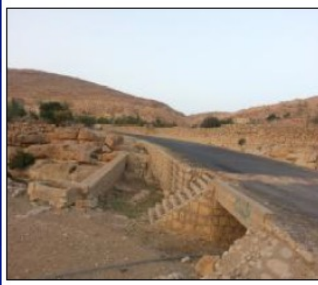
Water harvesting of road runoff, side drains and culvert into small pond, Yemen (REF Abyad 2013)
