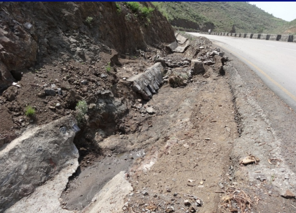
Erosion of side drains.
