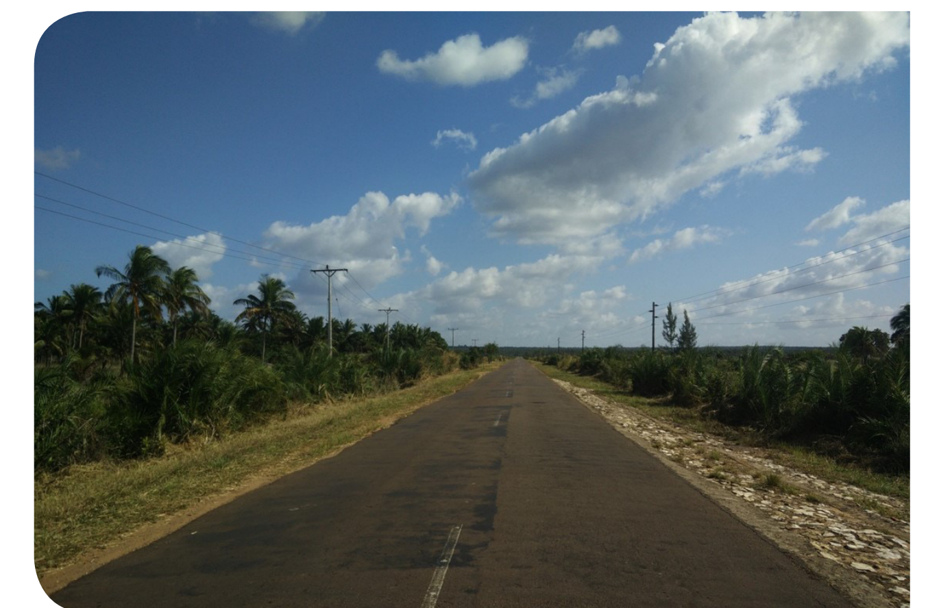
Low embankment road (mozambique) – saving costs and no uncontrolled floods
