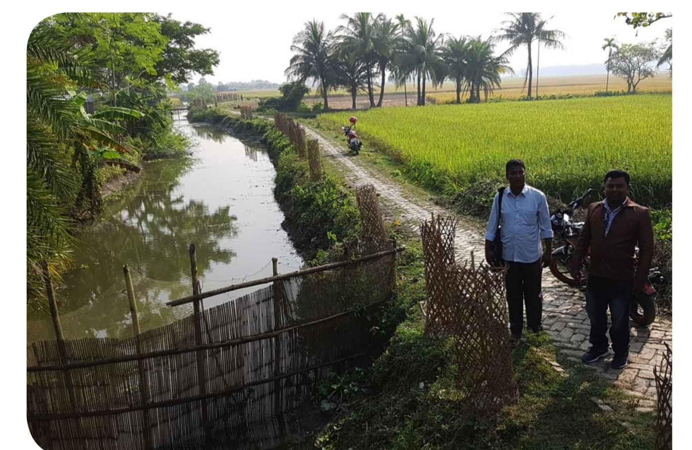
Creating storage and road levies in the flood prone plain (Bangladesh)
