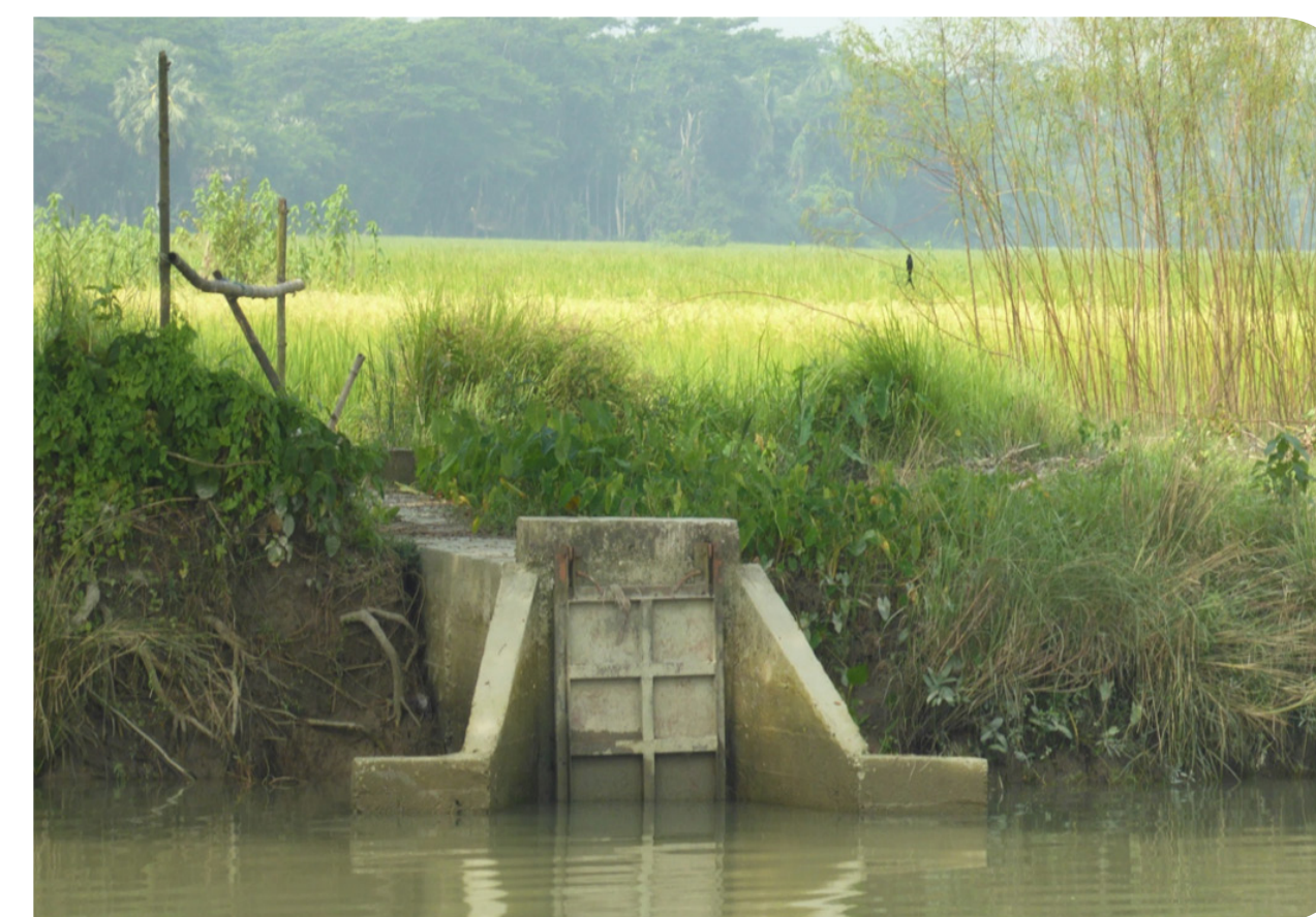
Managing water levels with gated cross drainage
