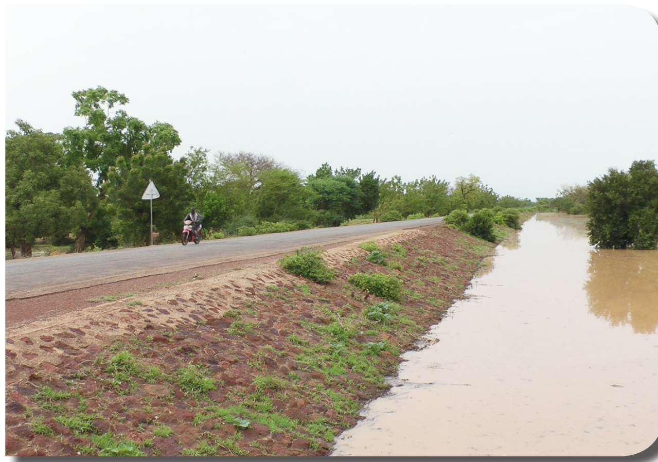
BURKINA FASO – WATER STORAGE WITH ROAD BODY
