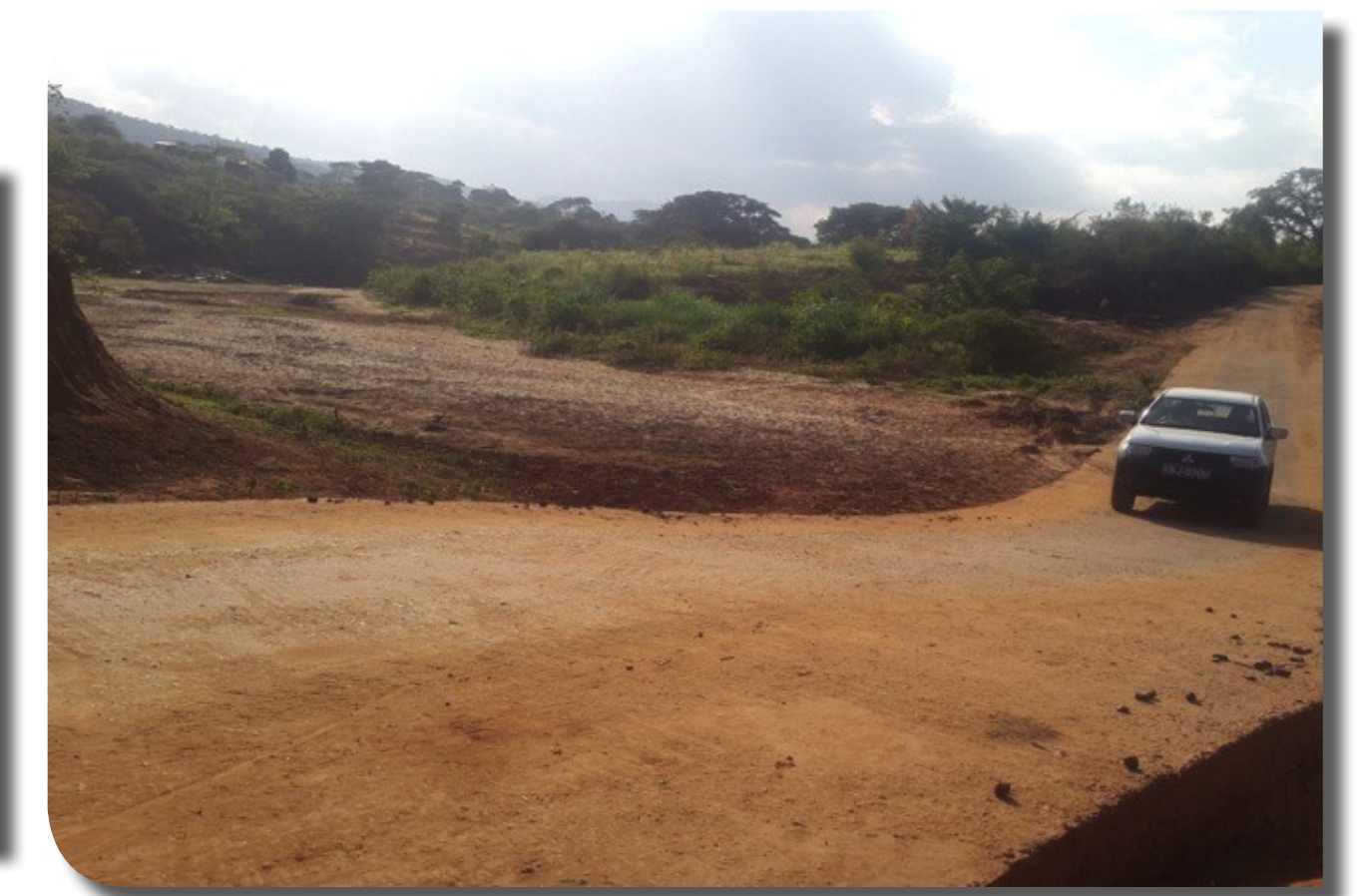
KENYA – ROAD DRIFTS FOR WATER RETENTION
