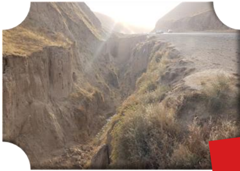
Erosion and sedimentation
