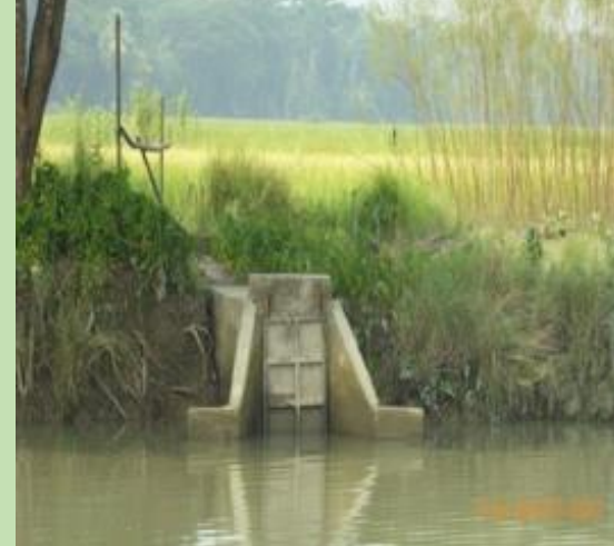
Gated culverts for water management
