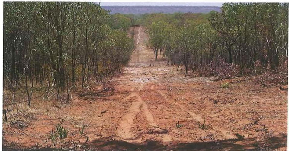
Plate 36. Poor site- long steep slope.
