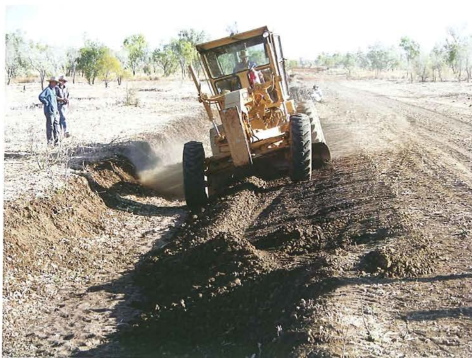
Plate 47. Battering off sides of a gully.
