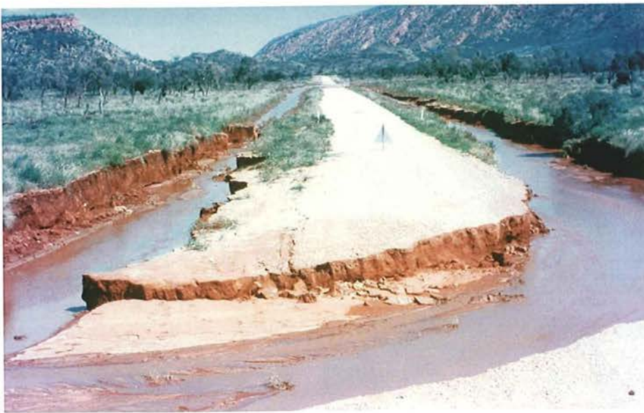
Plate 43. Gully erosion beside and across a road.
