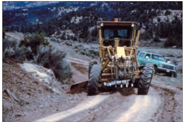
Photo V-3: Blading to maintain an insloped road template.
