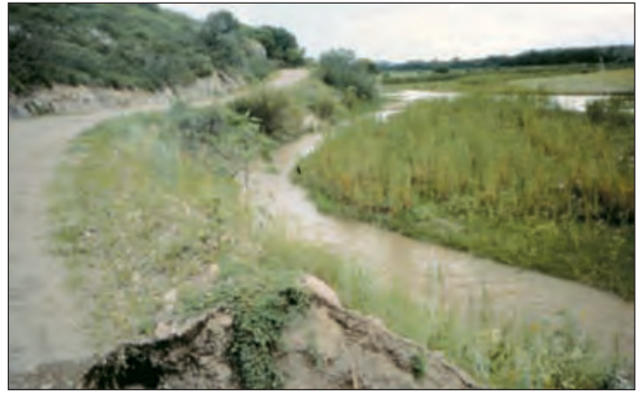
Photo VIII-4: Road encroachment on streambank.
