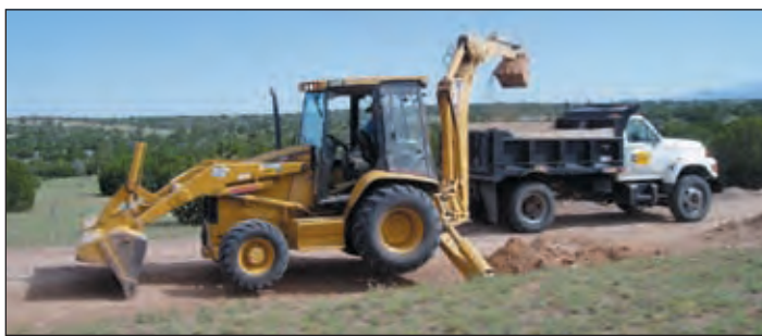
Photo IX-2: Backhoe removing sediment from a culvert inlet.
