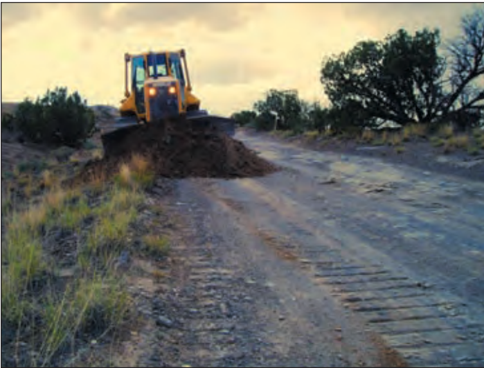
Photo V-4: Removing the unwanted berm will allow surface runoff to spill this outsloped roadway.
