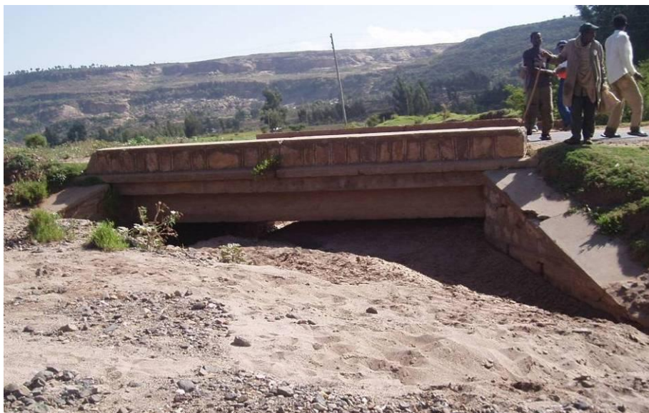
Figure 4-5 Small bridge in need of channel maintenance Wukro Agridat Zalambesa
