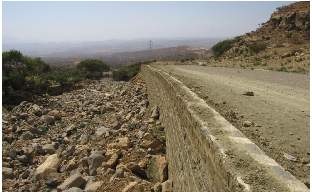
Figure 4-20 Bank stabilization and river protection Mekel-Abi Adi-Adwa km 71+9
