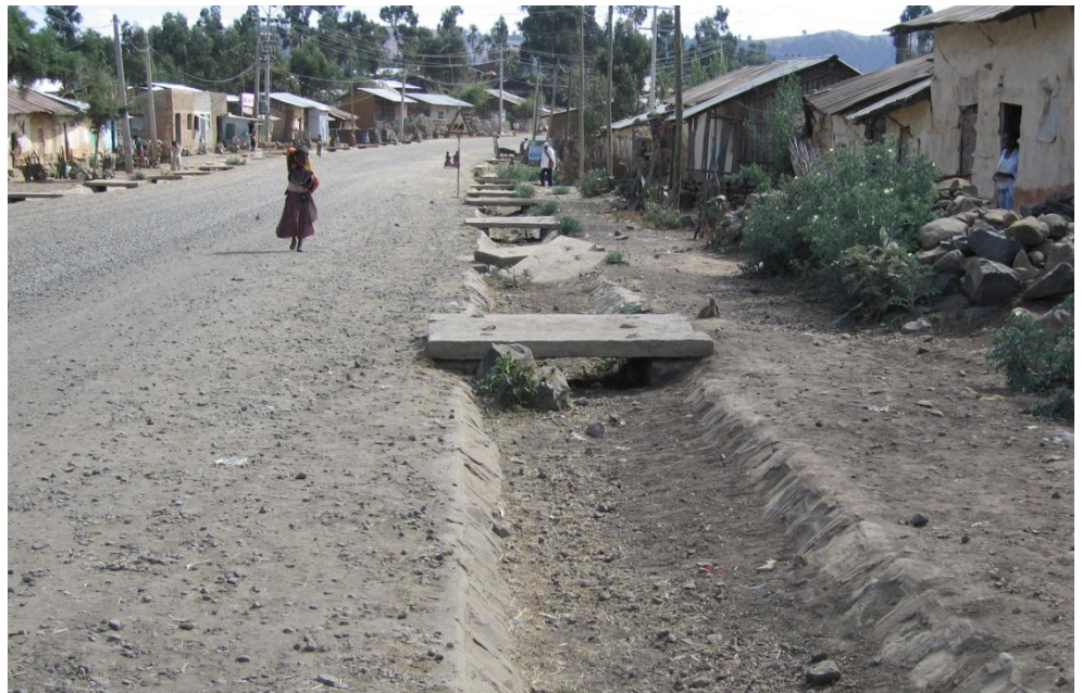
Figure 4-24 Roadside ditches filled with sediment through town section Hagera Salam
