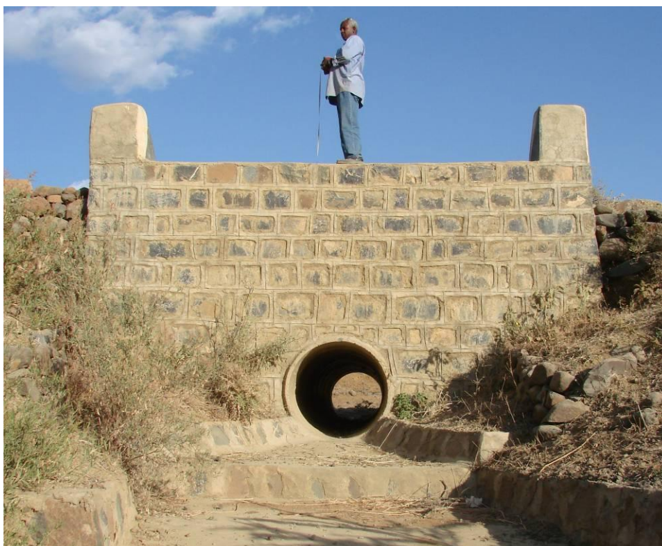
Figure 3-5 Concrete pipe culvert Mekele - Abi Adi- Adwa road
