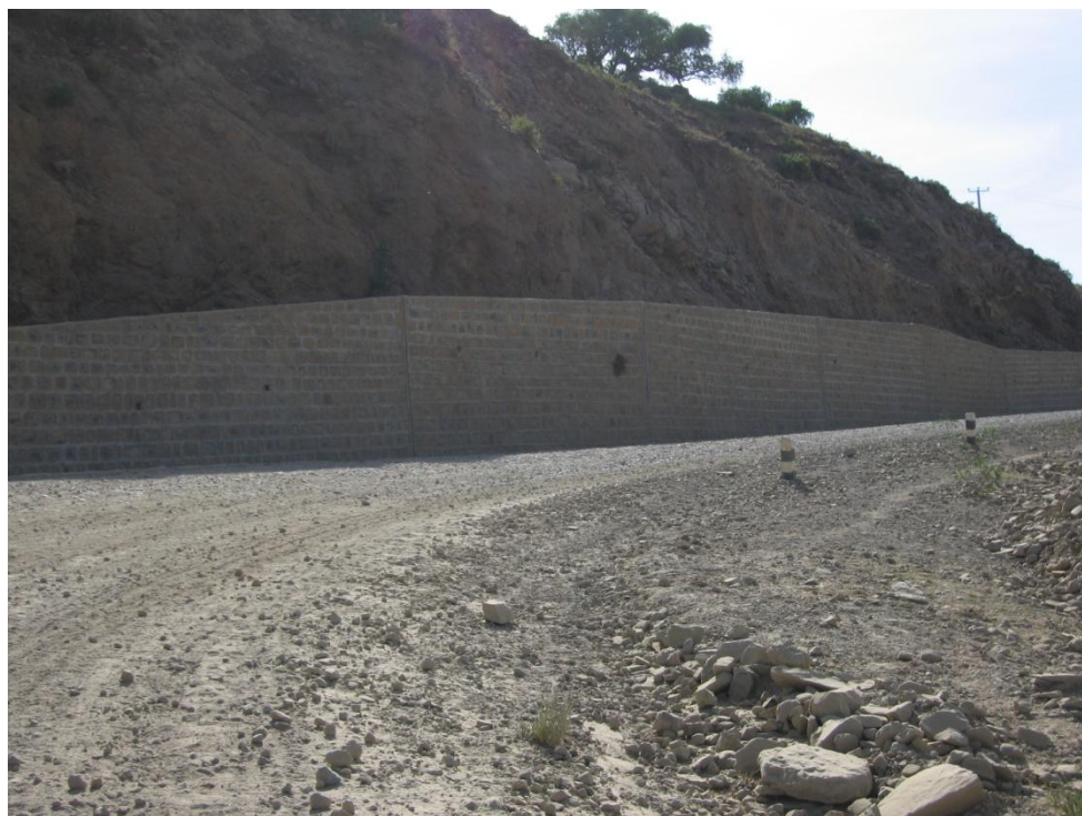
Figure 4-17 Rockfall protection retaining wall Mekele-Abi Adi-Adwa km 52+3
