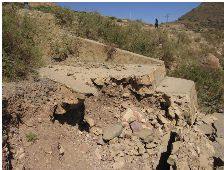
Figure 4-10 Eroded culvert outlet protection Mekele-Adwa km 39+038
