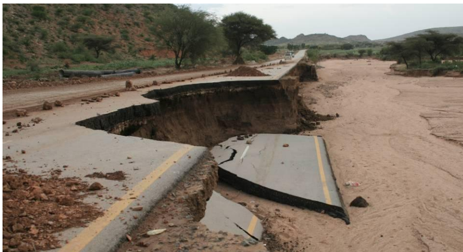
Figure 4-21 Roadside erosion Dire Dawa Region
