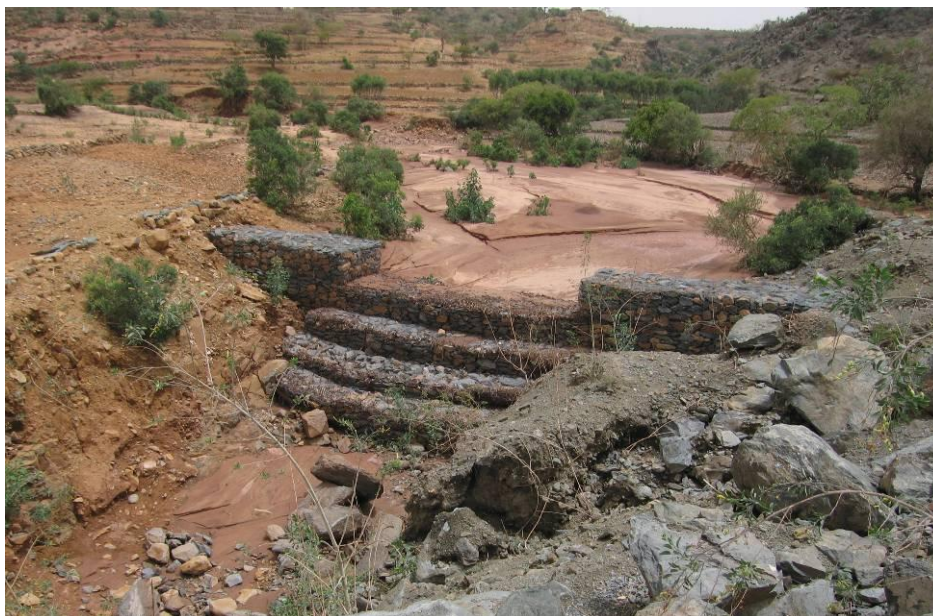
Figure 4-4 Large scale river works effort using rock gabions Mekele-Adwa
