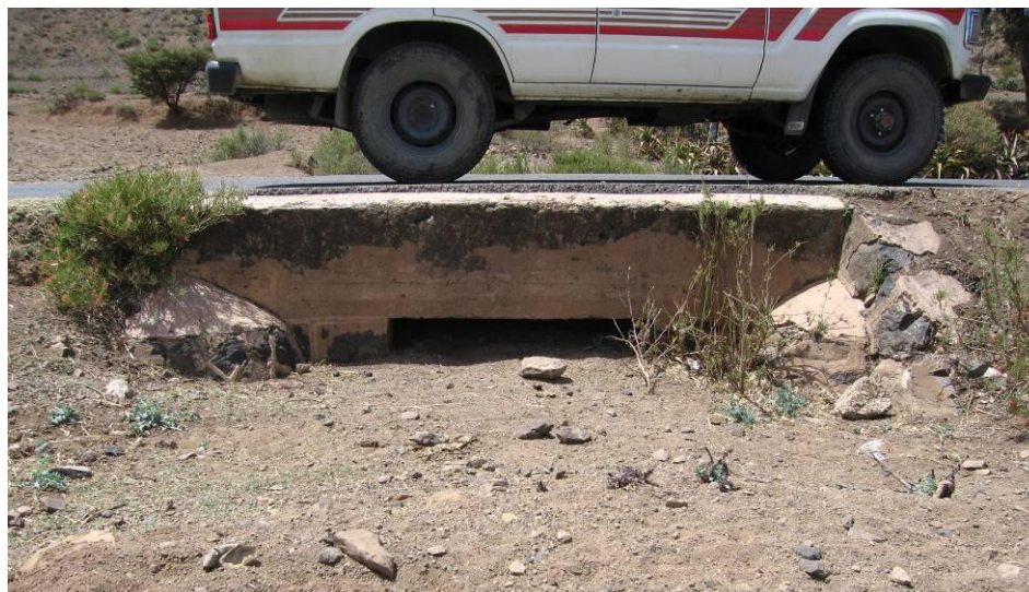
Figure 4-7 Slab culvert filled with sediment Wukro Agridat Zalambesa
