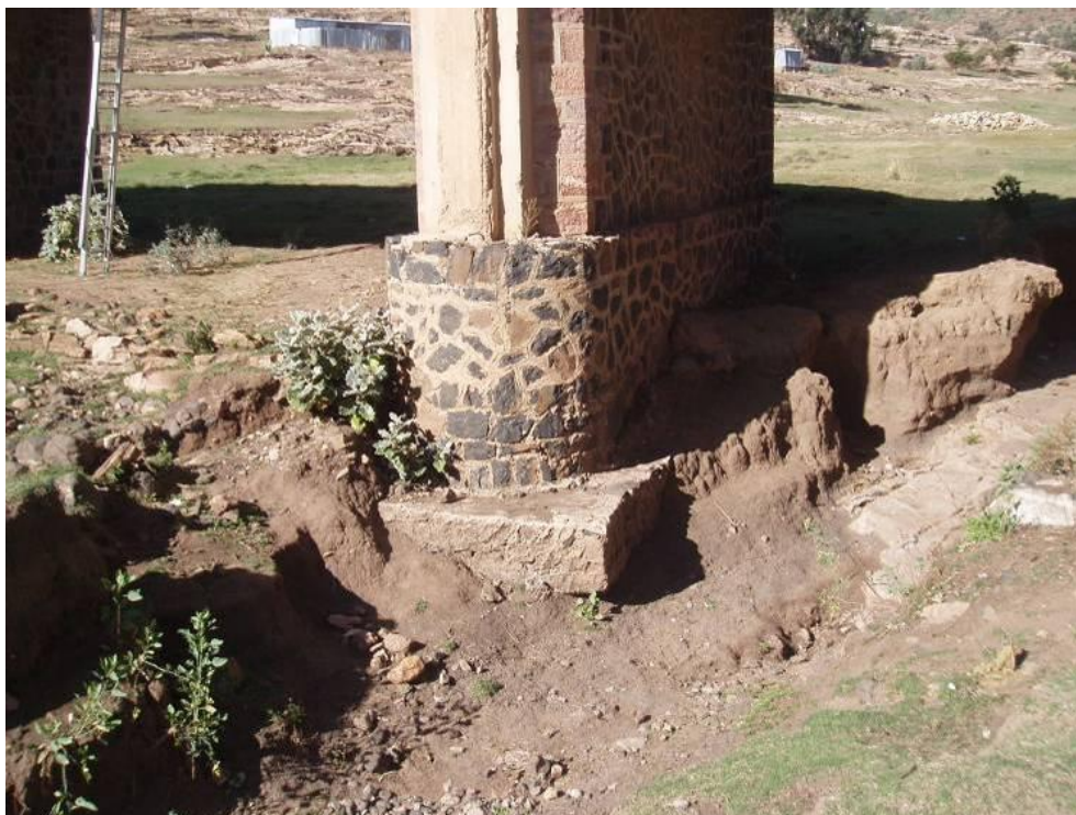
Figure 4-3 Local bridge scour Wukro Agridat Zalambesa road
