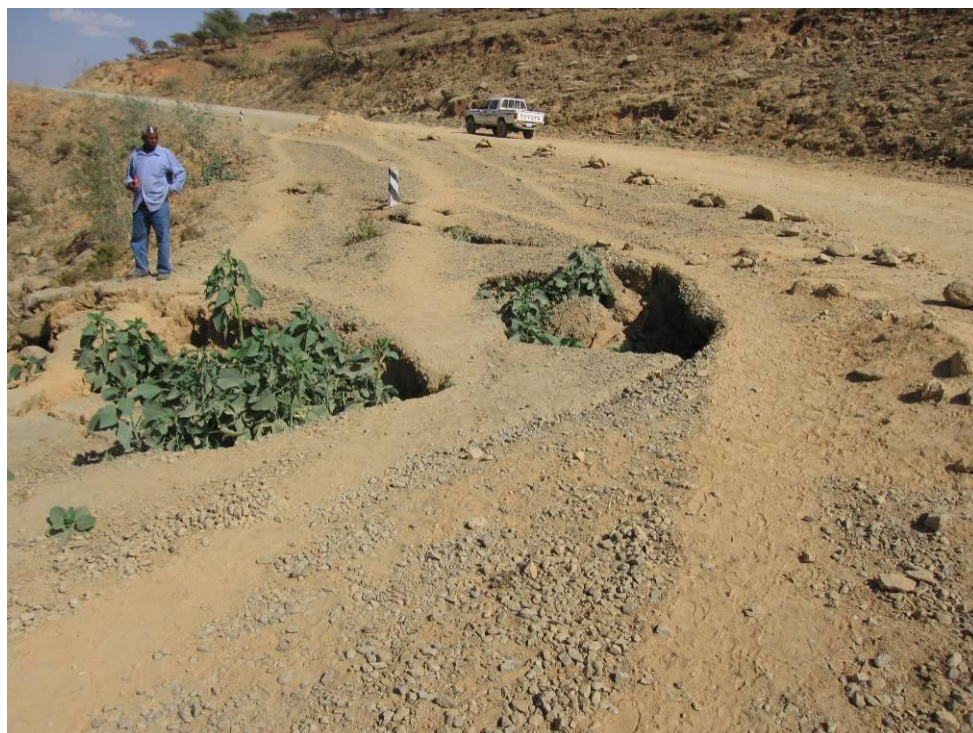
Figure 4-16 Small slip landslide Mekele-Abi Adi-Adwa km 115+800
