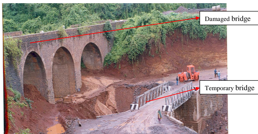
Figure 5-2 Temporary bridge installation in Ethiopia
