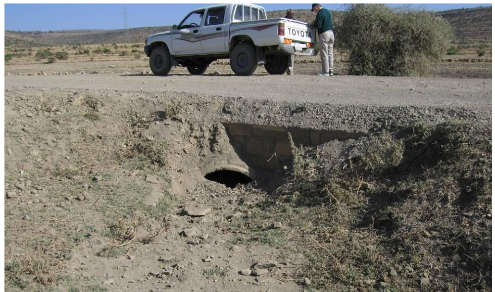
Figure 4-9 Pipe culvert filled with sediment Mekele-Adwa km 24+931
