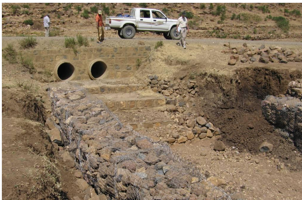
Figure 4-13 Increased culvert outlet protection Mekele-Adwa km 68+722
