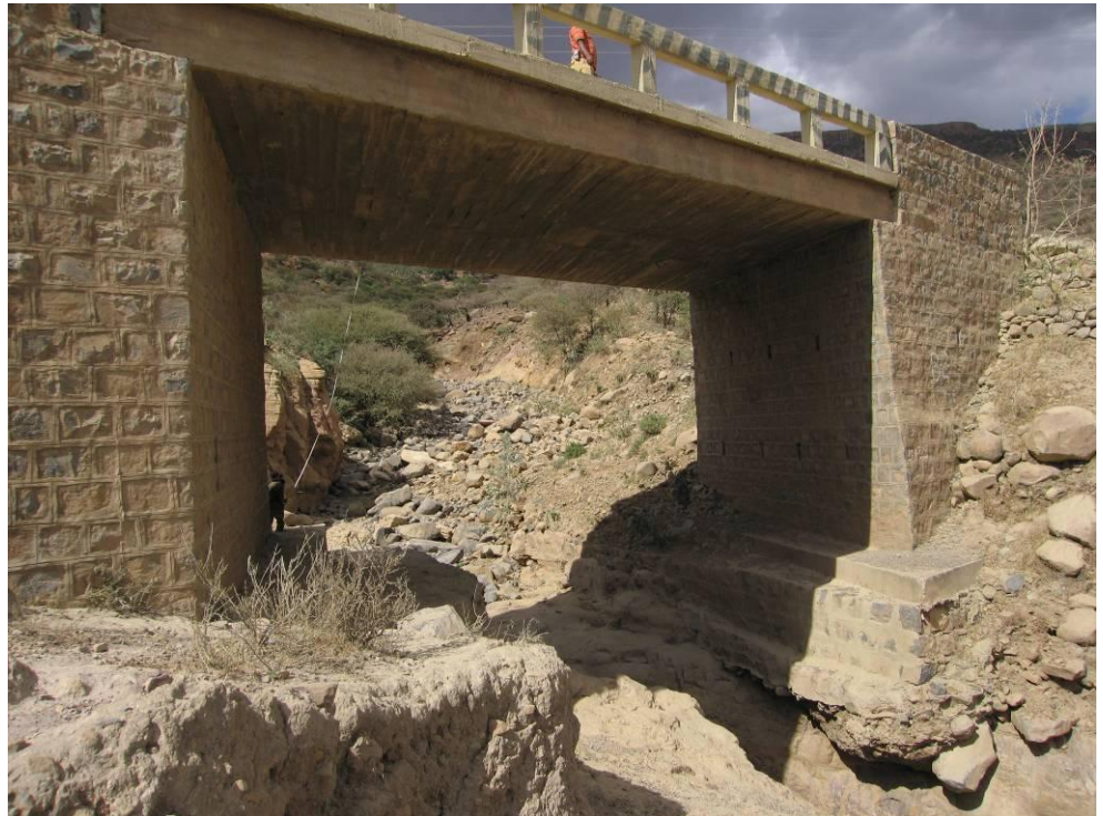
Figure 4-6 Bridge scour, Mekele Abi Adi Adwa road, km 73+685
