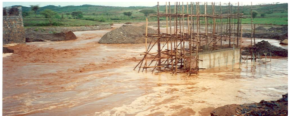
Figure 9-5 60 meter replacement bridge destroyed during construction, 2002 Road A-75
