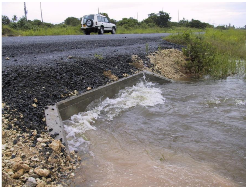
Figure 6-1 Example of inadequate culvert sizing when climate changes
