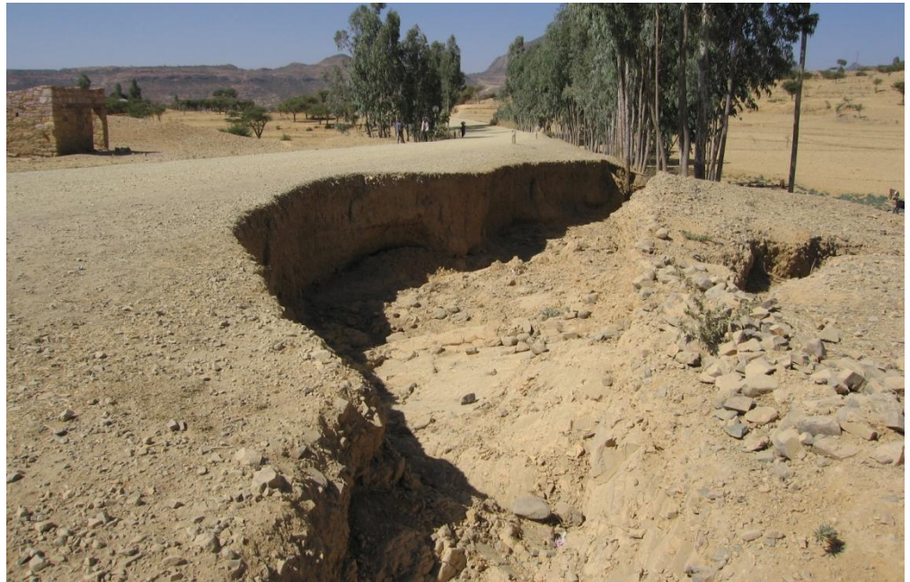
Figure 4-11 Diversion potential through gravel road Mekele-Adwa km 165+946
