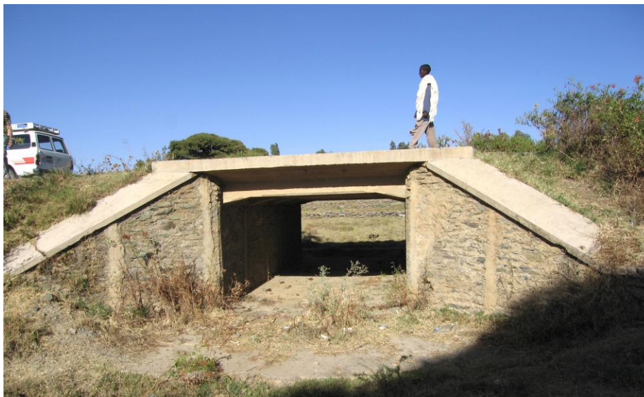
Figure 3-4 Slab concrete culvert Wukro Agridat Zalambesa road
