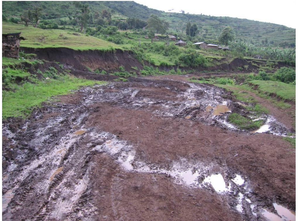
Figure 4-15 Poorly draining earth surface road, Uganda
