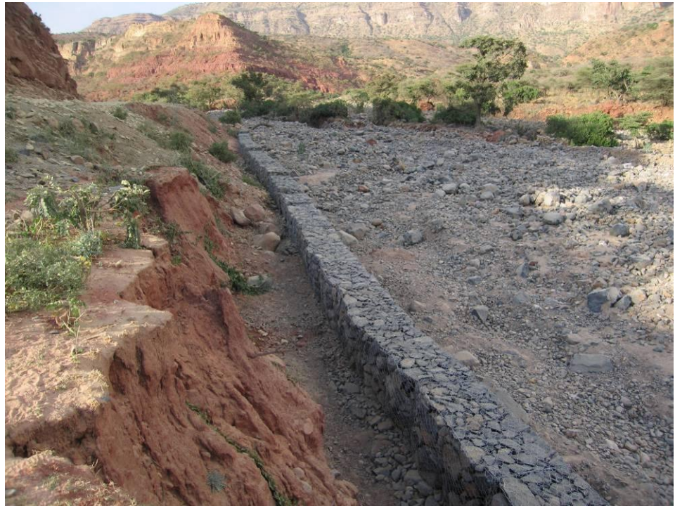
Figure 4-19 Gabions used as bank protection Mekele-Abi Adi- Adwa km 83
