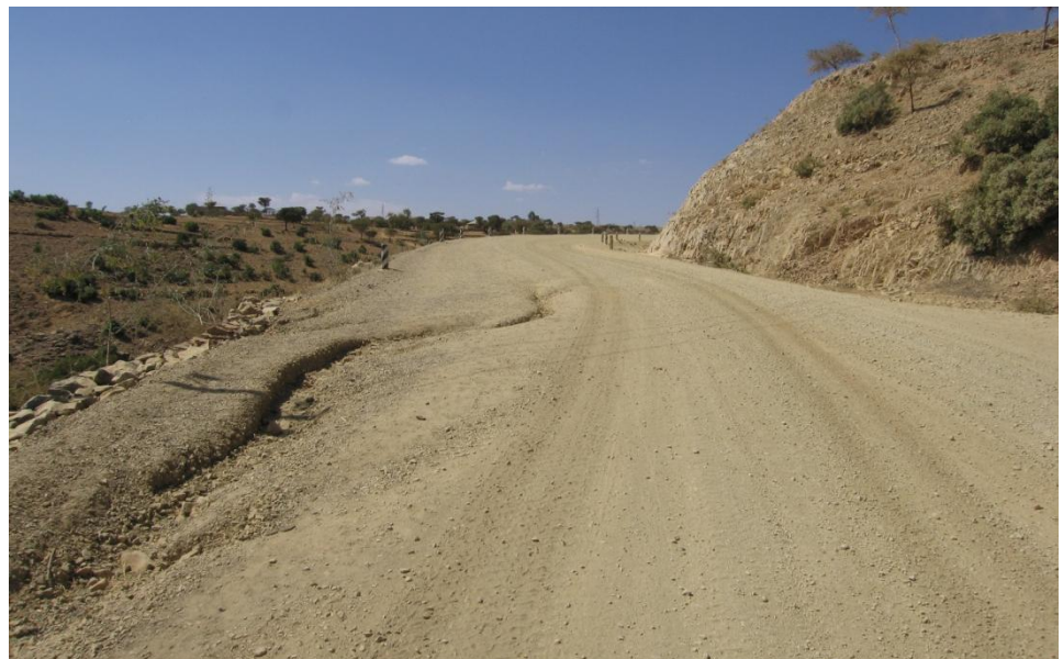
Figure 4-23 Poor surface drainage on gravel road Mekele-Adwa km 164+213
