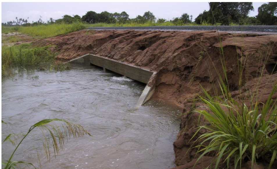
Figure 4-12 Road shoulder erosion caused from overtopping culvert with limited scour protection, Tanzania
