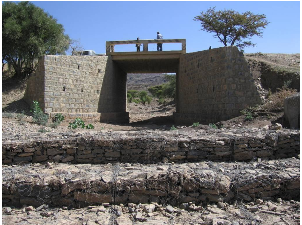
Figure 4-2 Downstream scour protection using gabions Mekele-Adwa km 156+751
