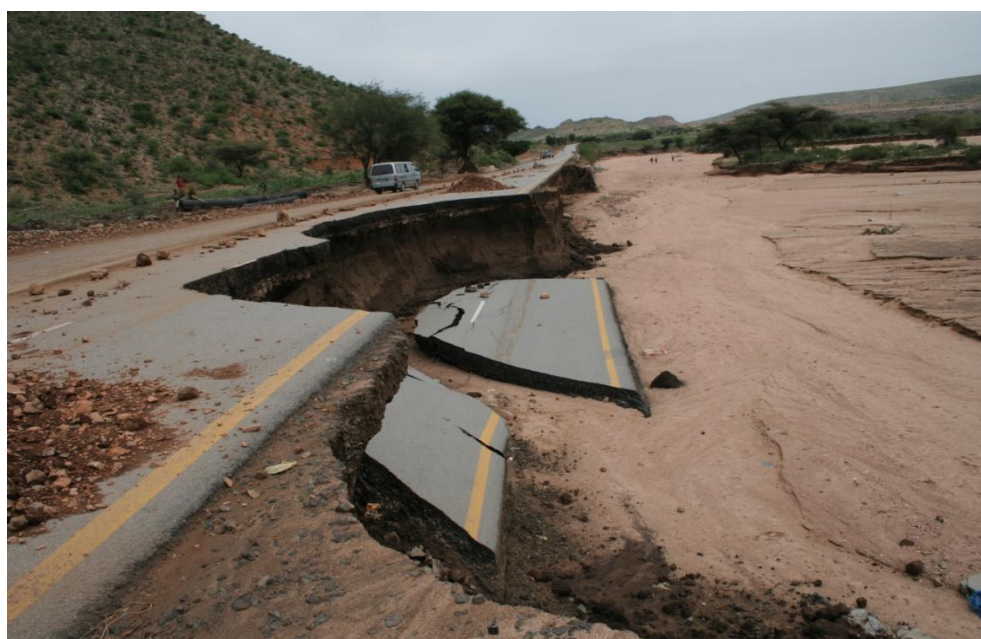
Figure 5-1 Road in Ethiopia partly washed away due to inadequate river bank protection
