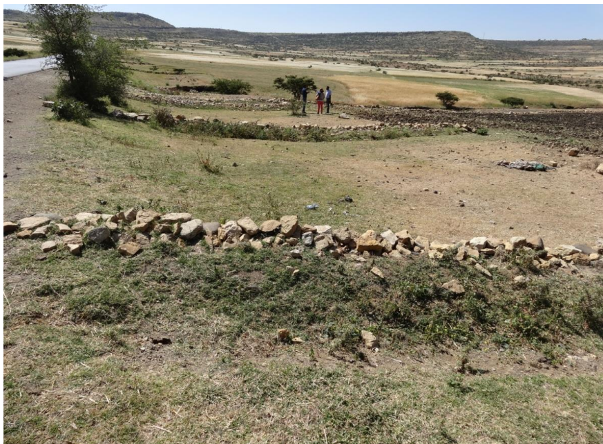
Figure 3a. Diverting roadside runoff into farm lands as part of moisture conservation in Kiken area (along Mekelle-Wukro road), Tigray, Ethiopia.
