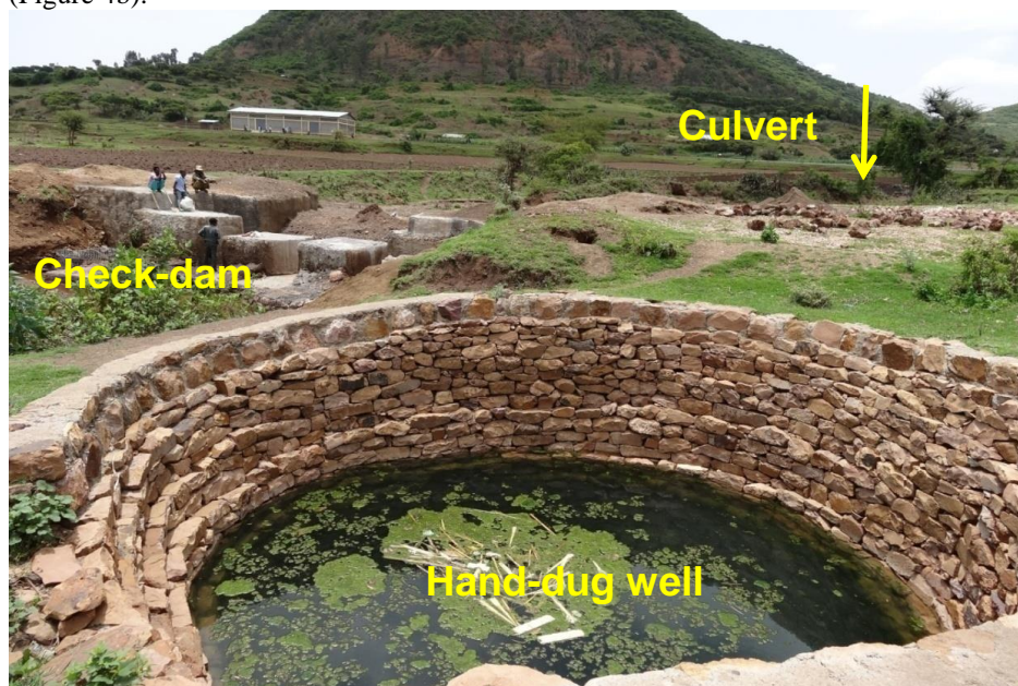
Figure 4a. Channelling water from a culvert into a check-dam is enhancing groundwater in Selekleka area, Tigray, Ethiopia.
