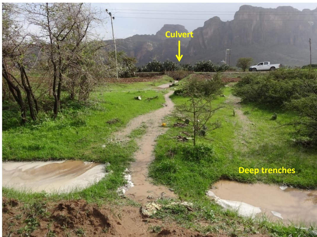
Figure 2a. Water from a culvert is channelled into a deep trenches in Megab area, Tigray, Ethiopia. Hand-dug well downstream of these trenches is used for monitoring.
