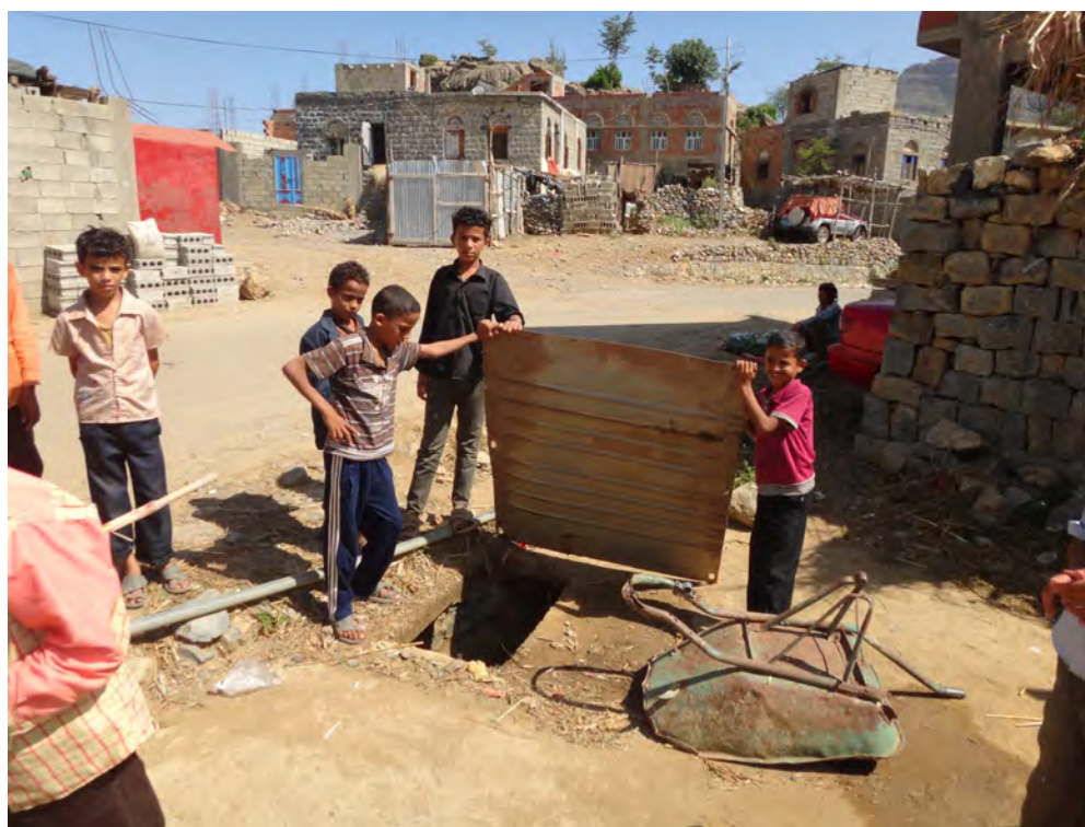
Water cistern filled by run-off from road-surface
