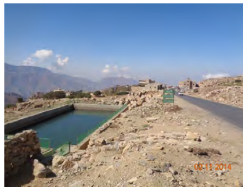
Road-run-off collected respectively from (up-slope) side drain and from escape in down-slope side drain
