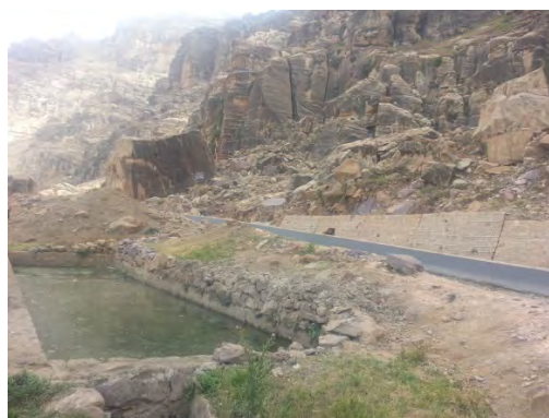
Pond storing spring water at down-slope (left) and spring water protection box up-slope (right)
