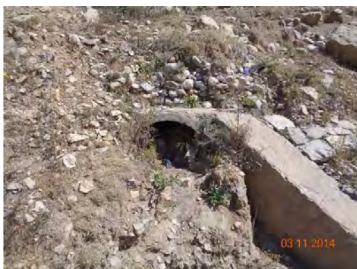
Blocked culvert inlets
