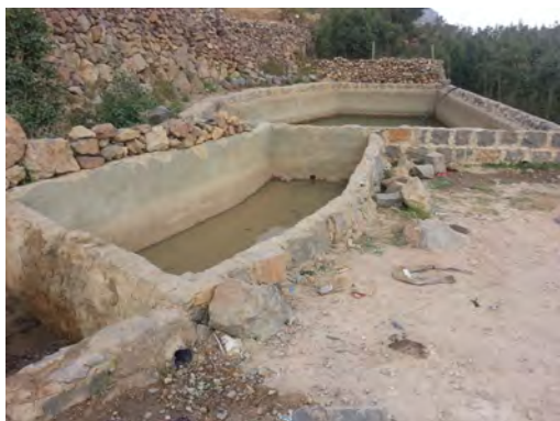
Ponds harvesting water from side drains
