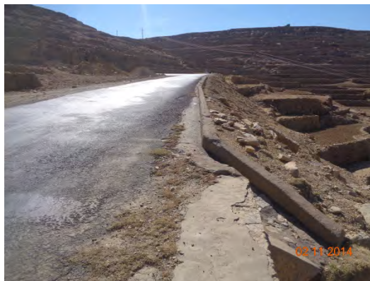
Erosion from uncontrolled run-off (left) and controlled road run-off (right)
