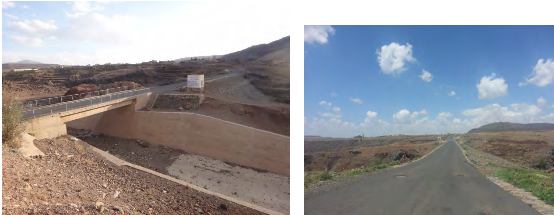
Figure #Road body as recharge dam in asphalt road
