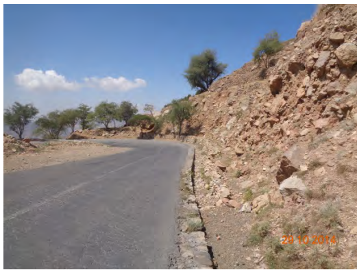
Road-run-off collected respectively from (up-slope) side drain and from escape in down-slope side drain
