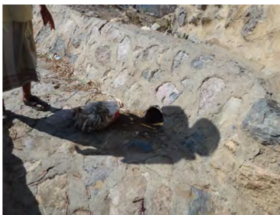
Cistern filled from road recharge and stone blocking first flush, Al Wastah
