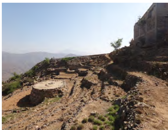
Cistern filled from road recharge and stone blocking first flush, Al Wastah
