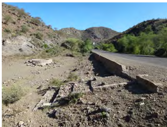
Flood water spreader from roads (left) and stepped intake (right)
