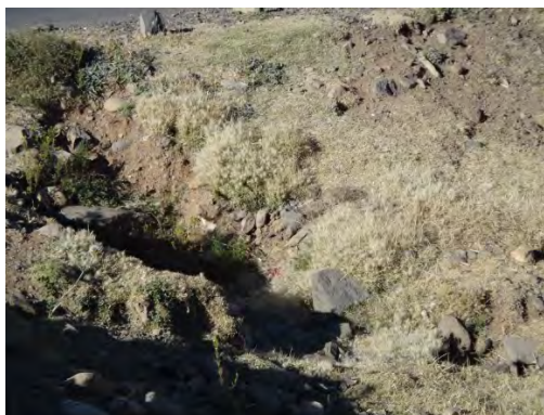
Erosion from uncontrolled run-off (left) and controlled road run-off (right)
