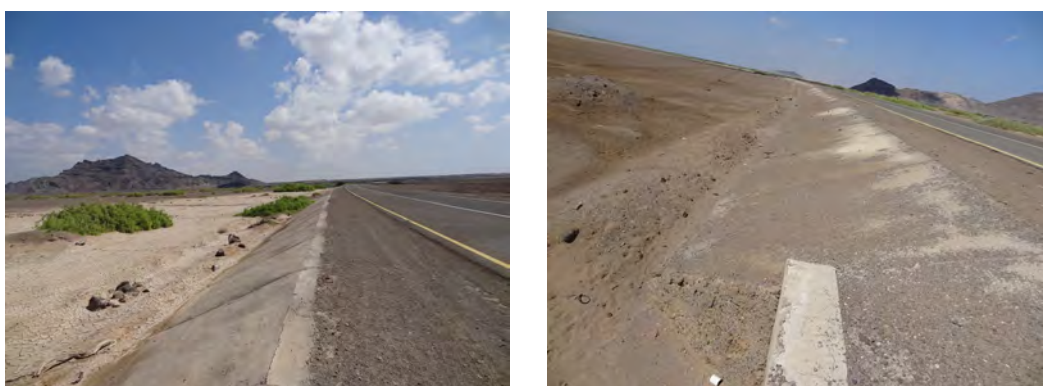
Figure # the embankment were protected by concrete and there is a small temporary bund to retain the water in the upstream (the potential is using gates in the culverts inlets).
