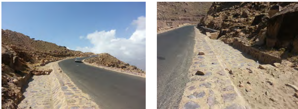
Figure # temporary rock checks in a ripraped side ditch
