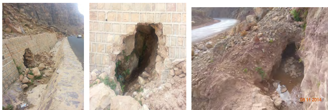
Figure #: Neglecting spring source requirements lead to land users to dig the retaining wall (picture at the middle and left) to follow the spring flow which disappeared after the road construction and hilll portection works. In other instances springs are re-excavated (picture on the right) after erosion
