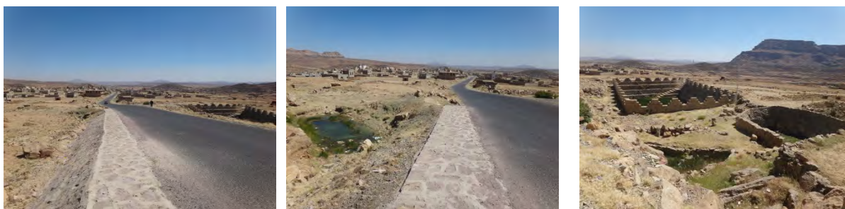
Figure #: Road embankment (left) interfere with base subsurface spring flow and the intercepted water by road embankment occurred in the other side (picture at the middle) of the spring flow point (picture at the right) thus by using clever road foundation this problem will be avoided.
