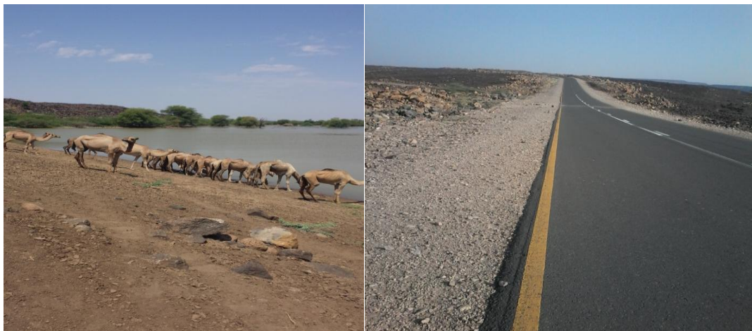
Figure . 3 Serdo kebele micro-dam constructed above the Asphalt road
