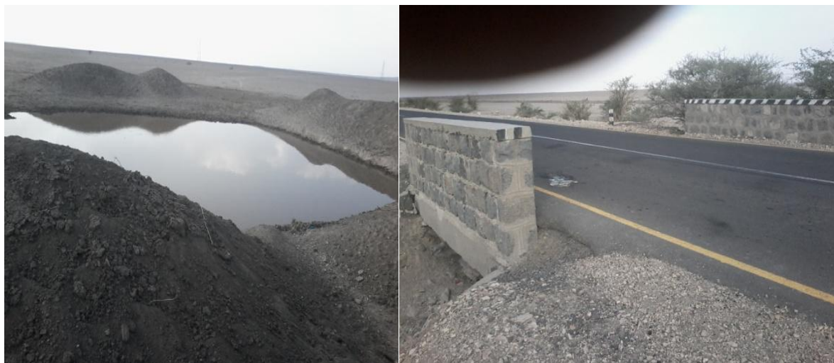
Figure 1. pond constructed along the main Ethio-Djibouti highway. Sordo kebele (Oct, 2015)
