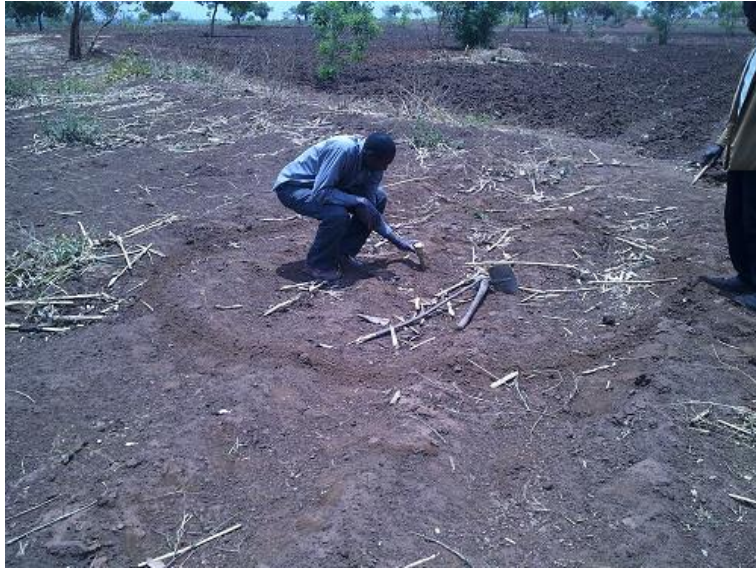
Marking out a Percolation Pond
