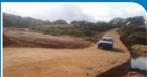
Kenya: Road crossing (non vented drift): retaining sand and water upstream which is used for brick-making, irrigation, and domestic use
