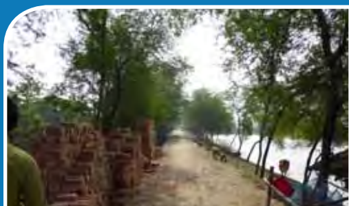
Bangladesh: Roads used for protection against river floods as well as for temporary storage of material and for road side grazing
