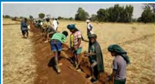
Ethiopia harvesting water from roads (1) creates additional water resources (2) reduces erosion, sedimentation and risk of flooding and waterlogging and (3) minimizes road damage
