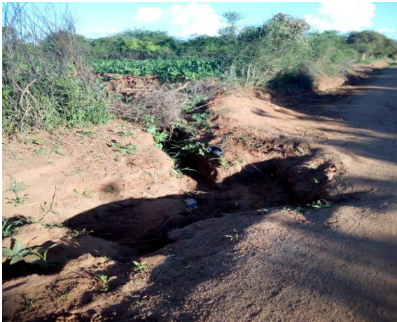
Figure 27: Mbiti diverts road water from culvert to his farm
