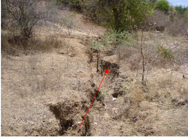
Figure 19: Gullying as a result of erosion by runoff from roads
