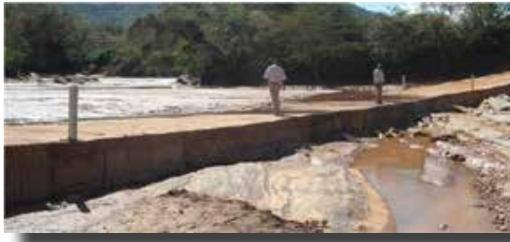
Figure 6: Non-vented drift crossing a river in Kenya
