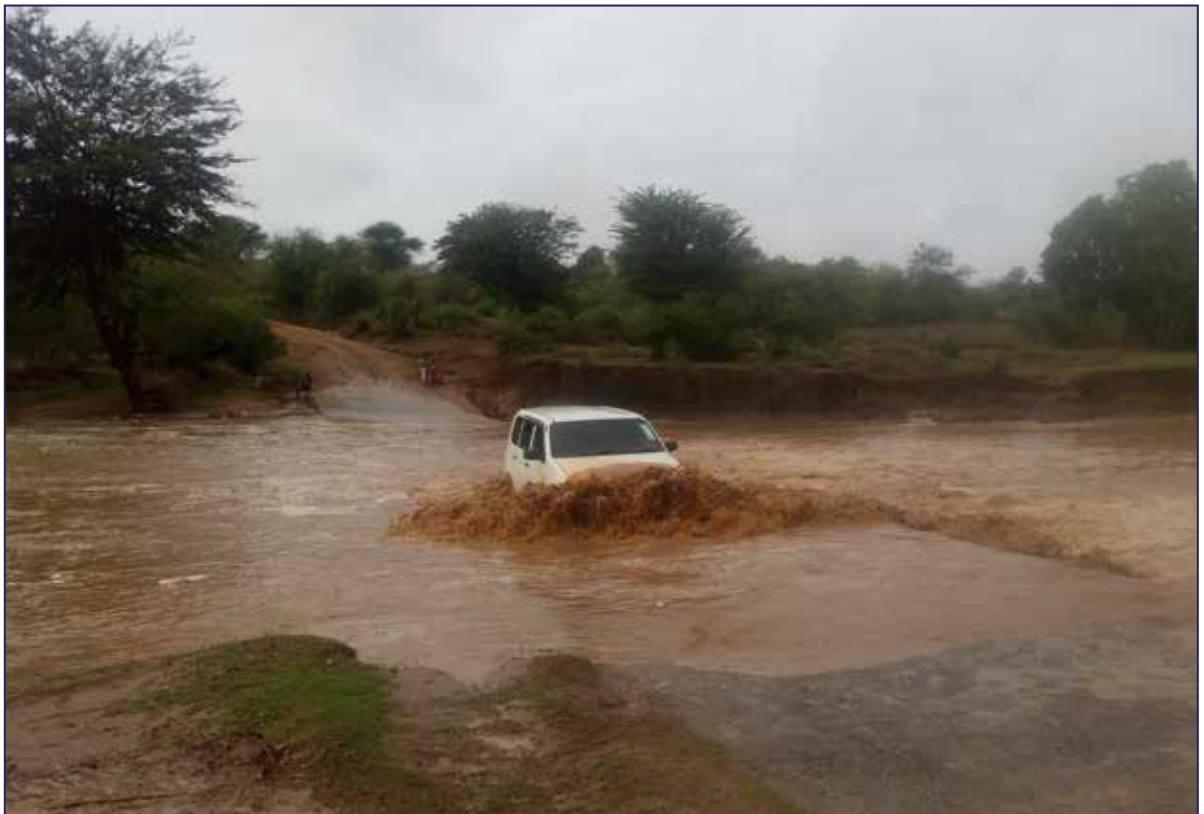
Figure 21: Passenger car passing on a non-vented drift when the flood is receding in Kitui, Kenya
