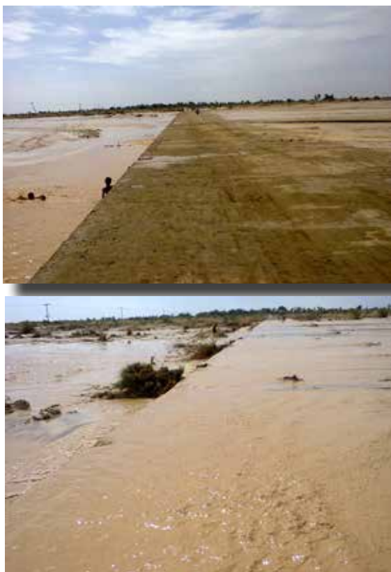
Figure 4: Road crossing at Kot Kaisrani (Pakistan), the upstream riverbed is stabilized with the construction of a drift
